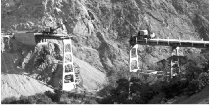
Construction at Anderson Reservoir, 1951
