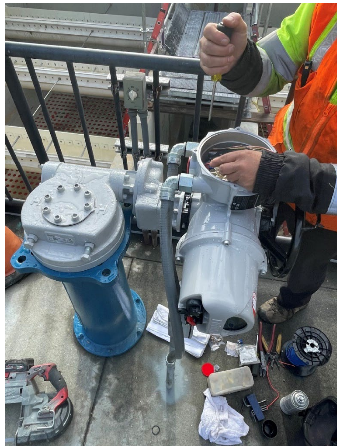
Installation of New Influent Valve, Deflector, and Actuator
