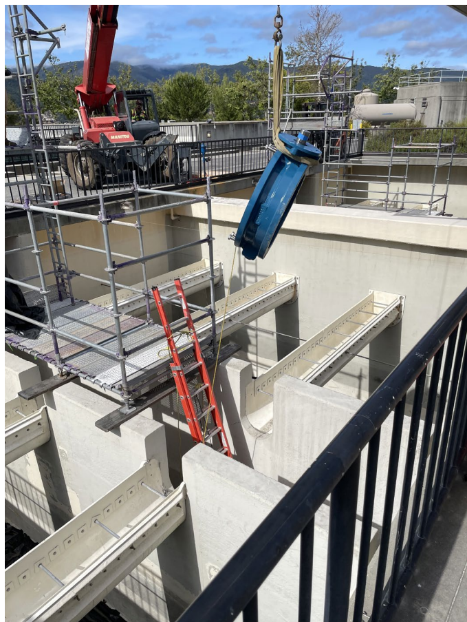
Installation of New Influent Valve, Deflector, and Actuator
