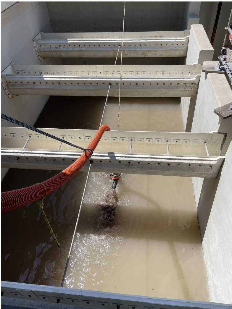
Installation of New Filter Media (Sand)
