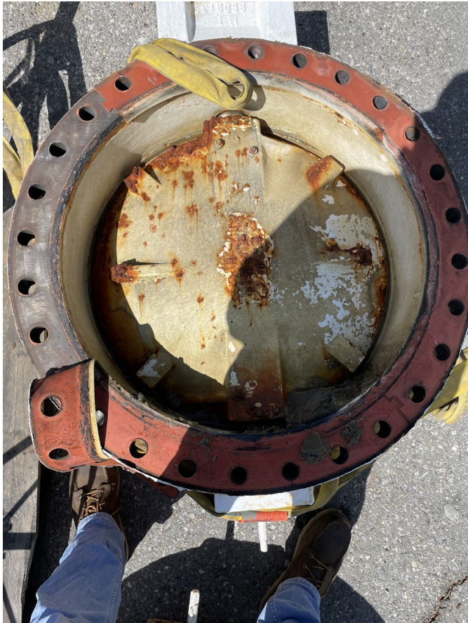
Removal of Existing Influent Valve, Deflector, and Actuator
