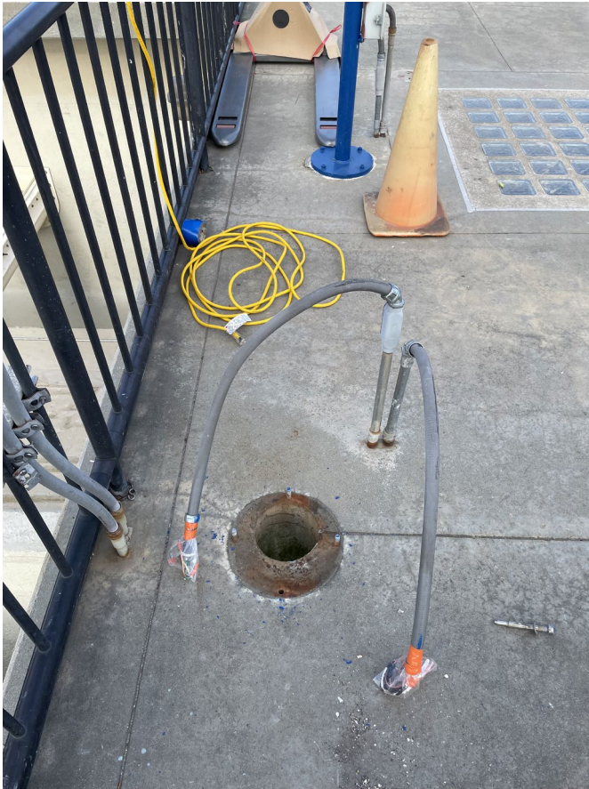
Removal of Existing Influent Valve, Deflector, and Actuator
