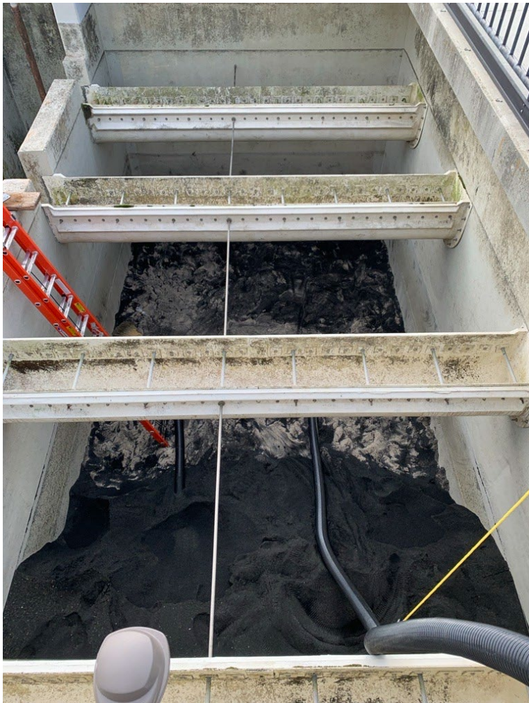
Removal of Filter Media – Granular Activated Carbon (Black) and Sand (Brown)
