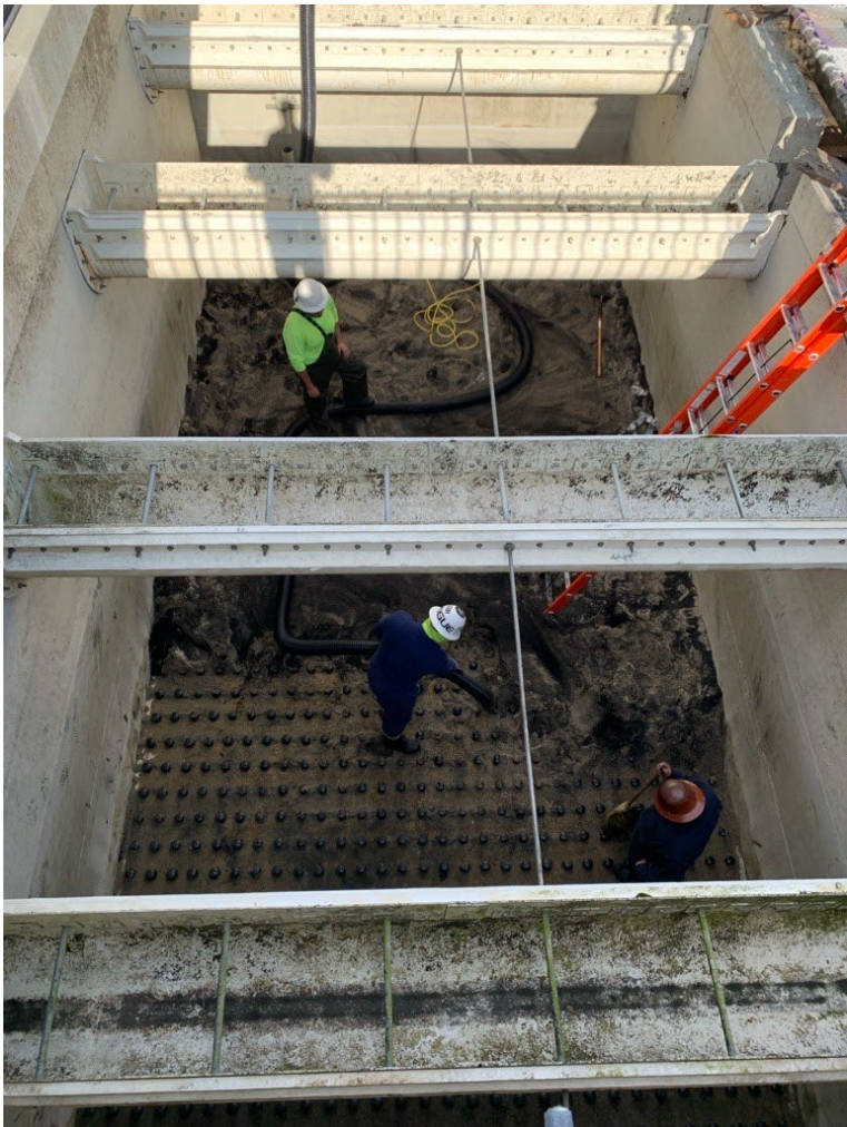
Removal of Filter Media – Granular Activated Carbon (Black) and Sand (Brown)
