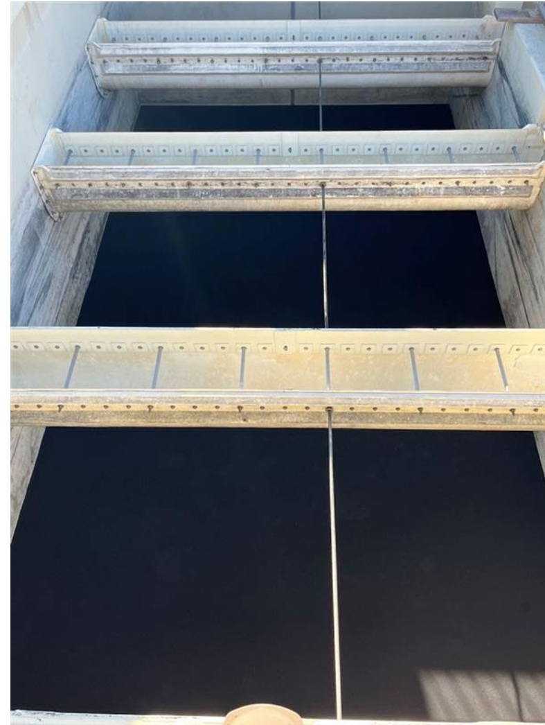
Installation of New Filter Media (Granular Activated Carbon)
