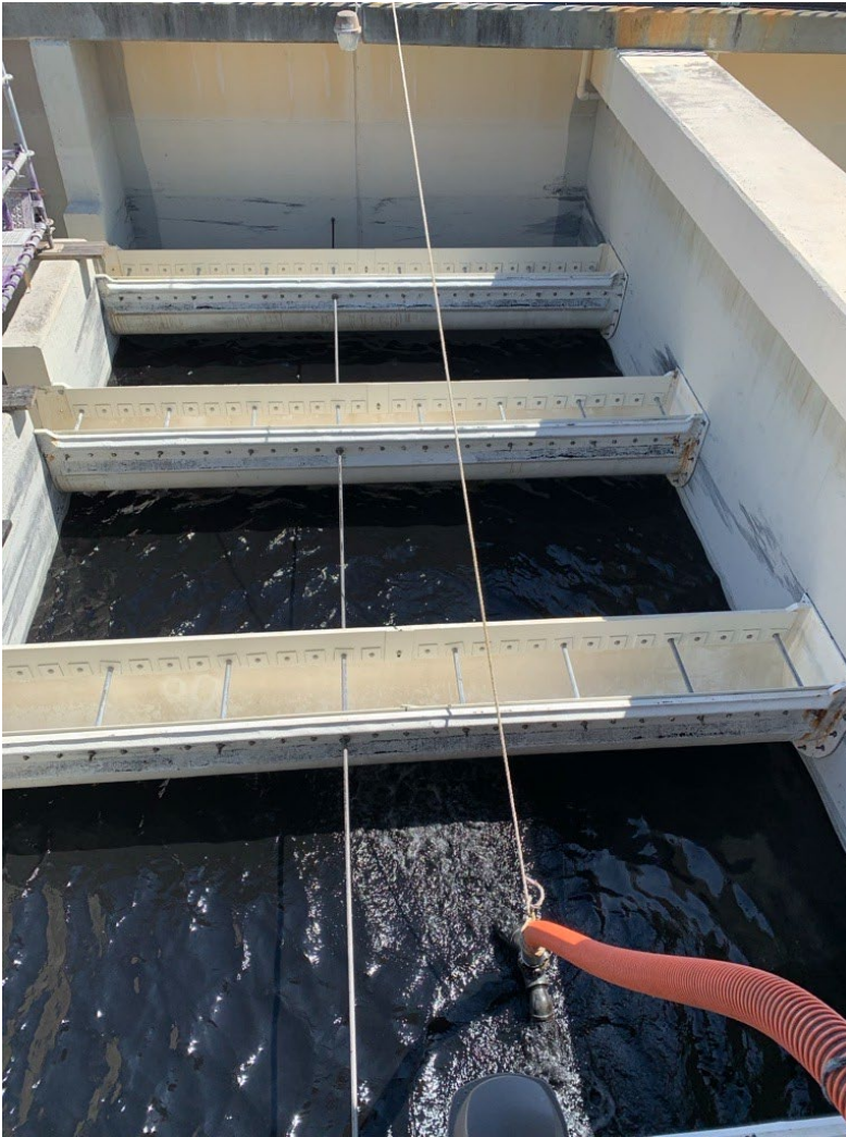
Installation of New Filter Media (Granular Activated Carbon)
