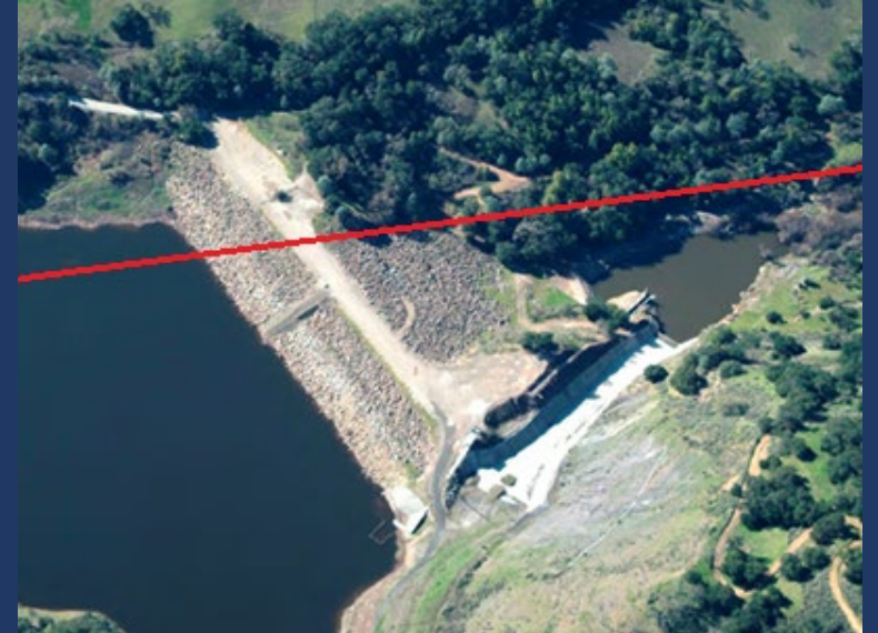
Calaveras Fault crossing embankment
