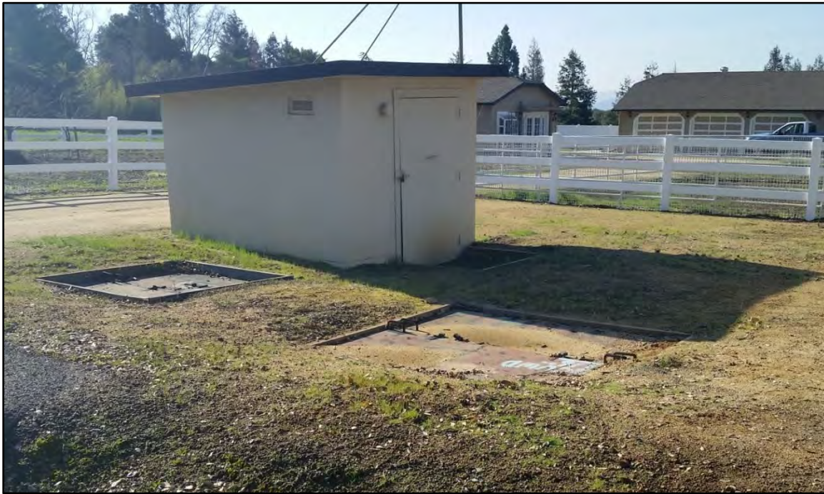
Photo 1. Existing chemical feed station located on Cochrane Road.
