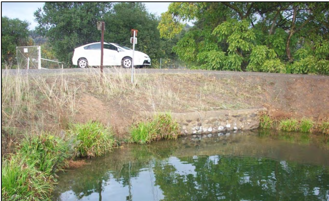
Photo 4. View of the Main Avenue Percolation Ponds in the southern portion of the project area where installation of the energy dissipater is proposed.
