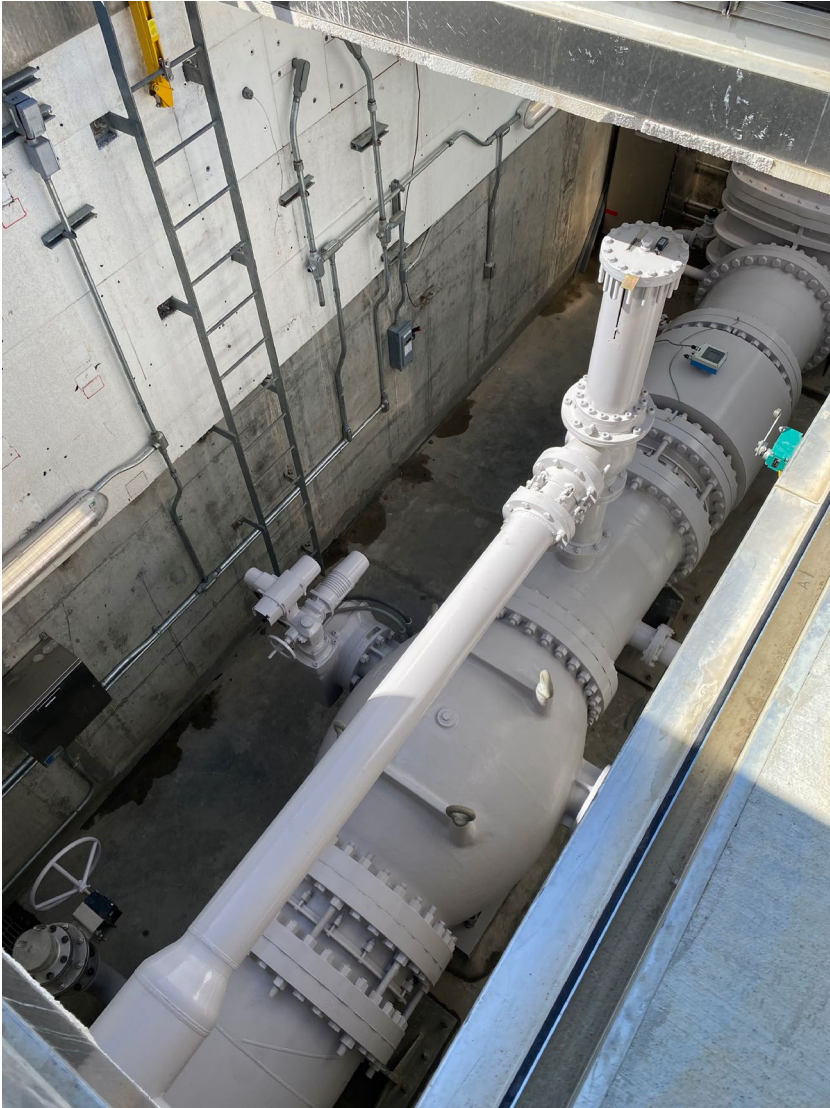
New Plunger Valve, Magnetic Flowmeter and Gate Valve
