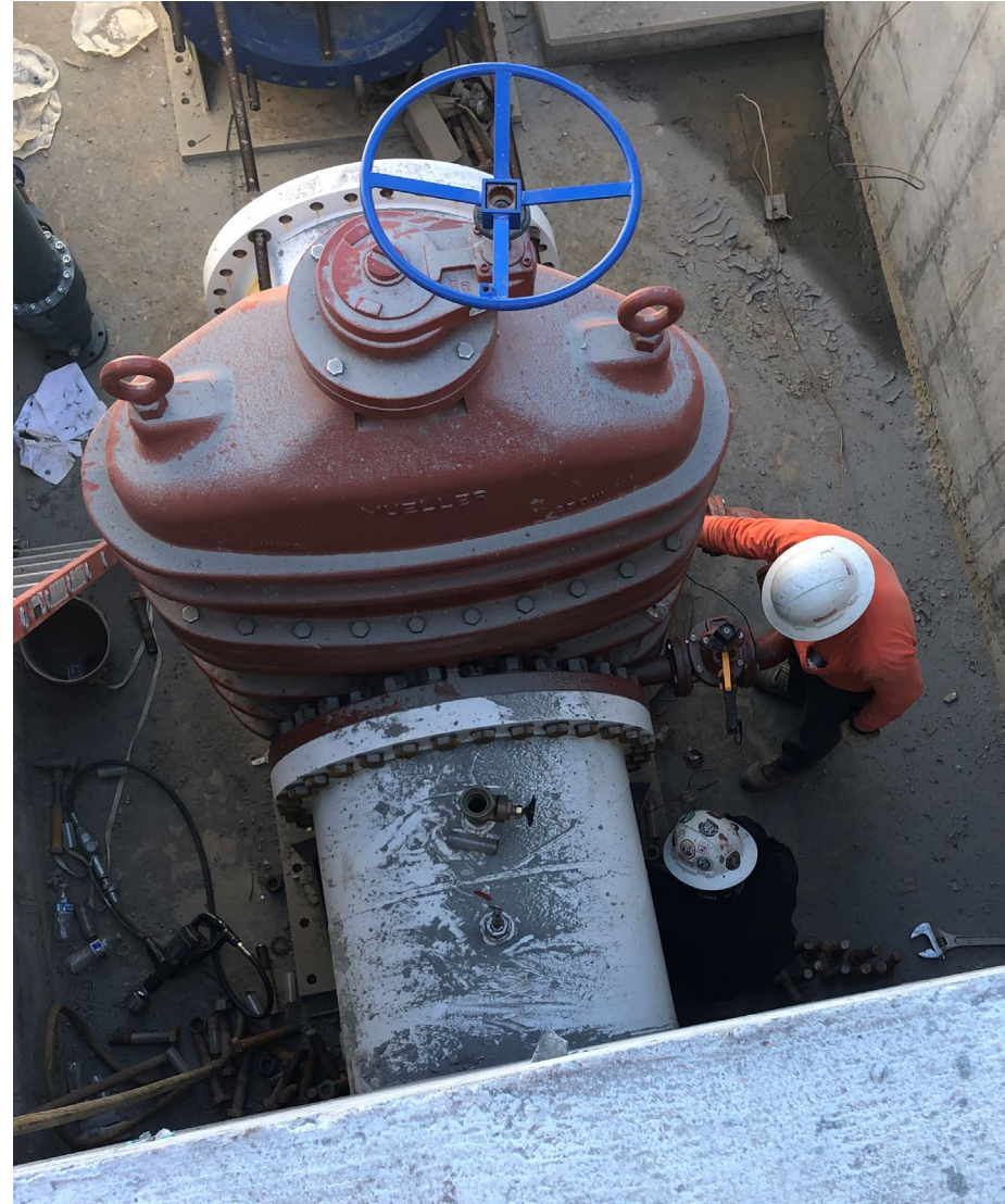
New Plunger Valve, Magnetic Flowmeter and Gate Valve
