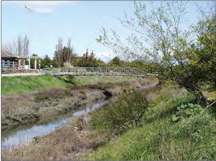
Permanente Creek, looking downstream at the golf course foot bridge
