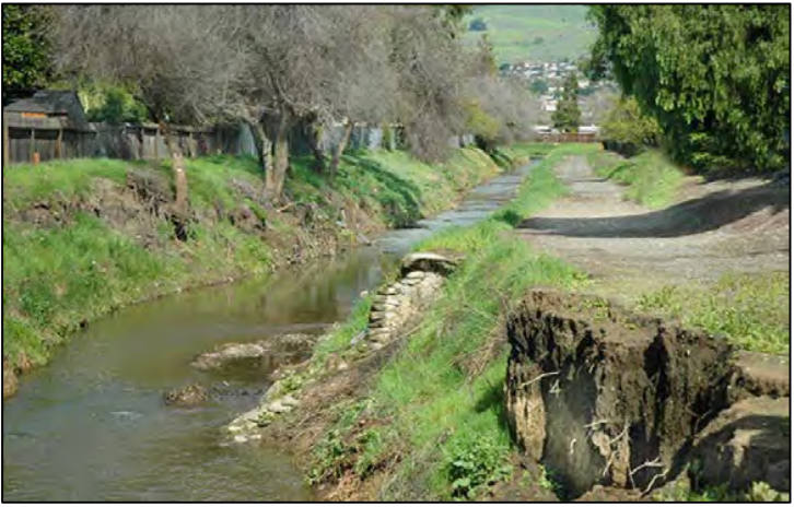
Lower Silver Creek looking upstream from Capital Expressway
