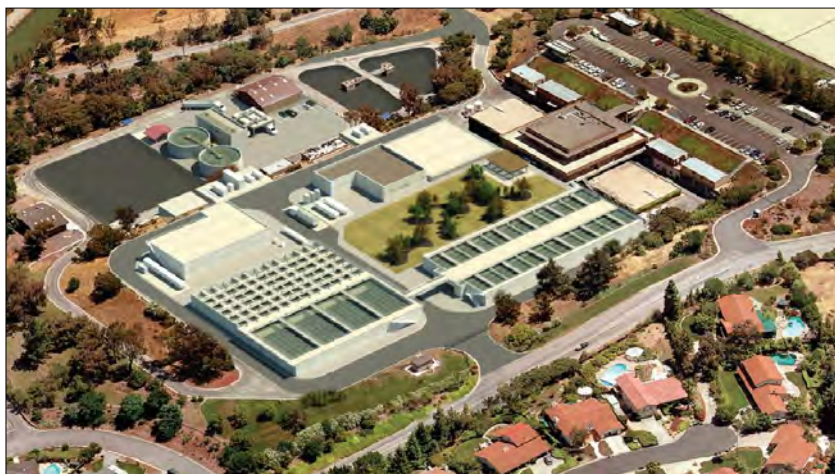
Artist rendering of the aerial view of the Rinconada Water Treatment Plant facing south after construction
