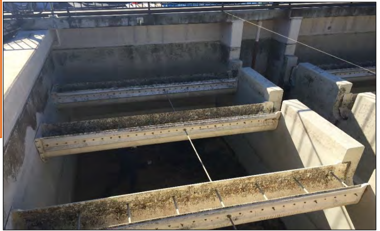
Santa Teresa Water Treatment Plant Filter Media Replacement
