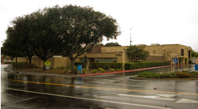
Existing Maintenance Building
