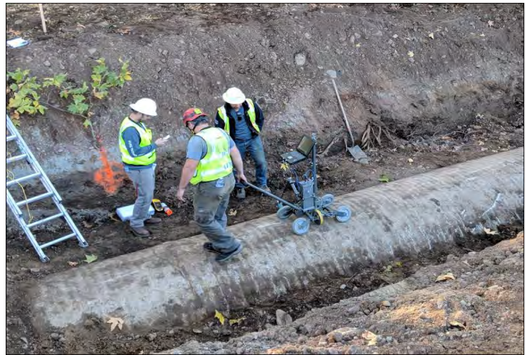
Almaden Valley Pipeline Replacement work is underway
