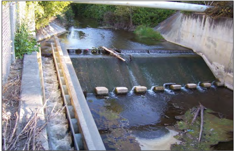
Example of a fish ladder to be modified or reconstructed for better fish passage
