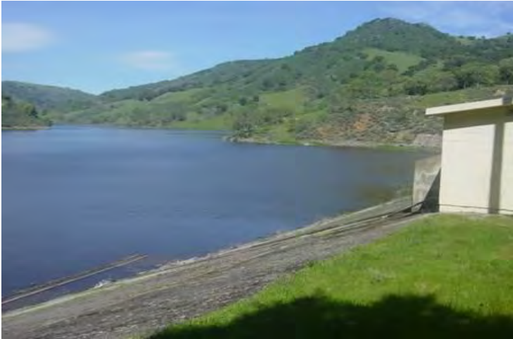
View of Pacheco Reservoir from the dam
