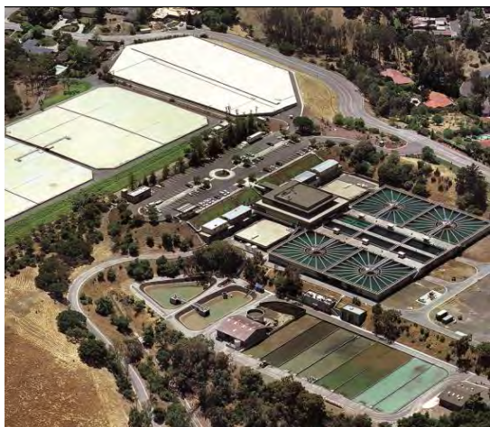
Aerial view of the Rinconada Water Treatment Plant facing west
