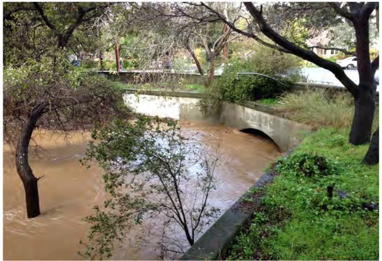
Upstream face of Pope/Chaucer Street with water surface approximately two feet below the soffit
