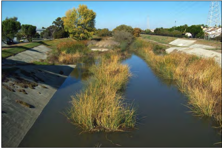
Lower Penitencia Creek, looking downstream from Milmont Drive
