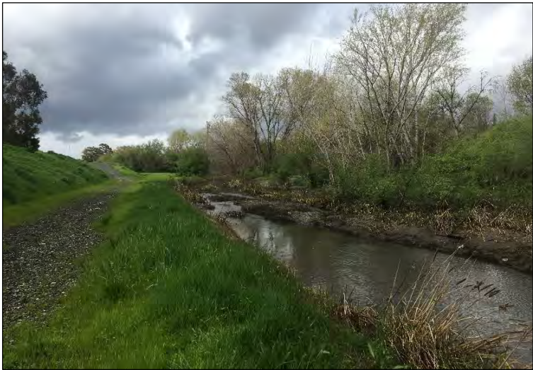
East bank of the Guadalupe River, looking upstream toward Trimble Road.
