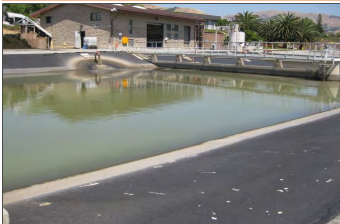
Existing settling pond and residuals building to be replaced with new residuals management facility
