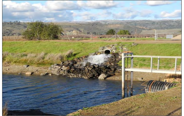
Madrone Pipeline Outlet into Madrone Channel looking North along Northbound Interstate 101
