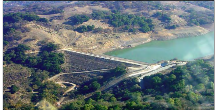
Aerial view of the Guadalupe Dam, spillway, and part of the reservoir
