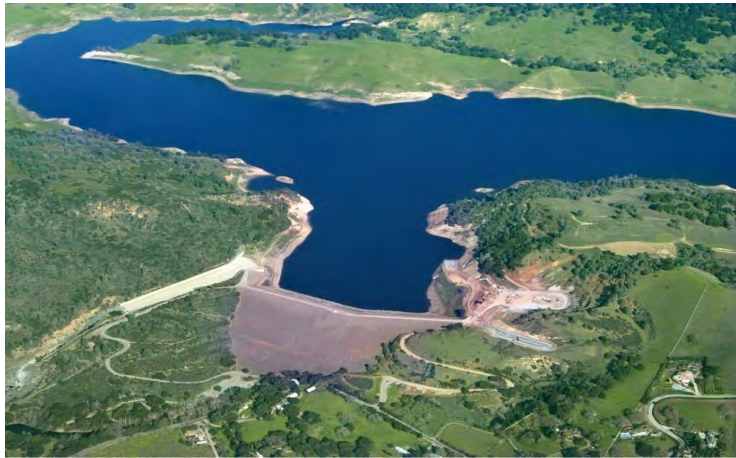
Aerial view of Anderson Dam and spillway, with a portion of the reservoir
