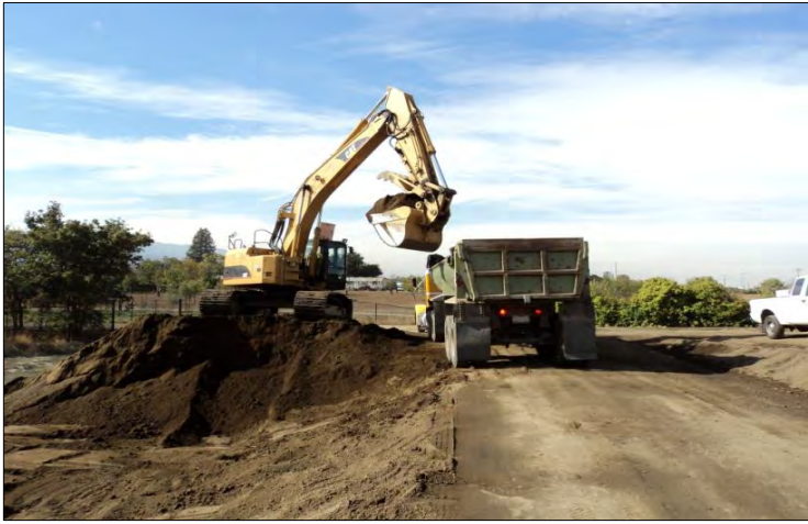
Sludge pond sediment removal at Santa Teresa Water Treatment Plant
