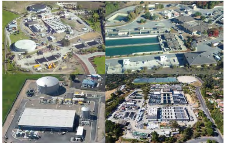
WTP Implementation Project
