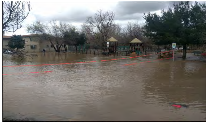
February 2017 flood event, on Rock Springs Drive looking northeast towards Rocksprings Park
