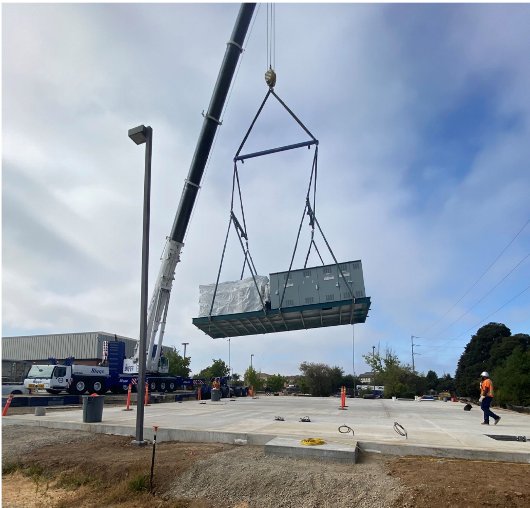
Secondary Unit Substation placed on foundation August 2025
