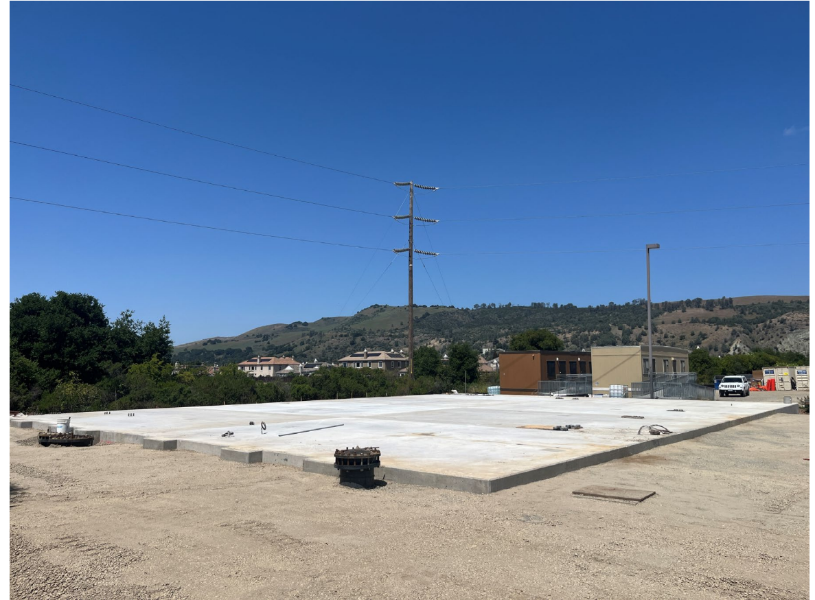
Concrete foundation slab completed in March 2025
