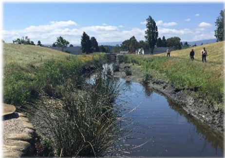
Sunnyvale West Channel
