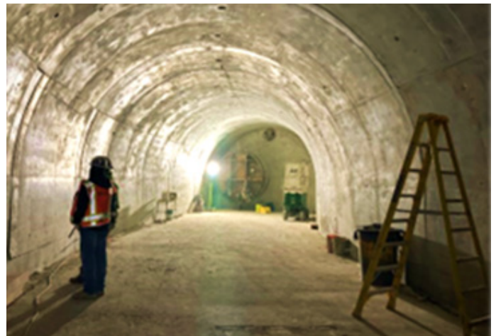
Anderson Dam Seismic Retrofit Project Completion of Pipeline Extension, February 2026
