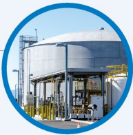
Silicon Valley Advanced Water Purification Center
