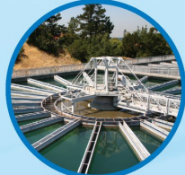
Rinconada Water Treatment Plant
