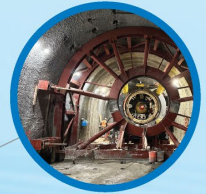
Anderson Dam Tunnel and Seismic Retrofit Projects
