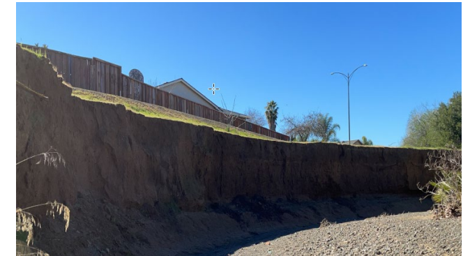
Thompson Creek Erosion – AMP
