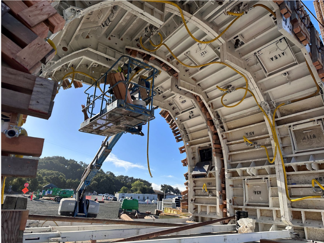
October 2024 Concrete formwork for mockup
