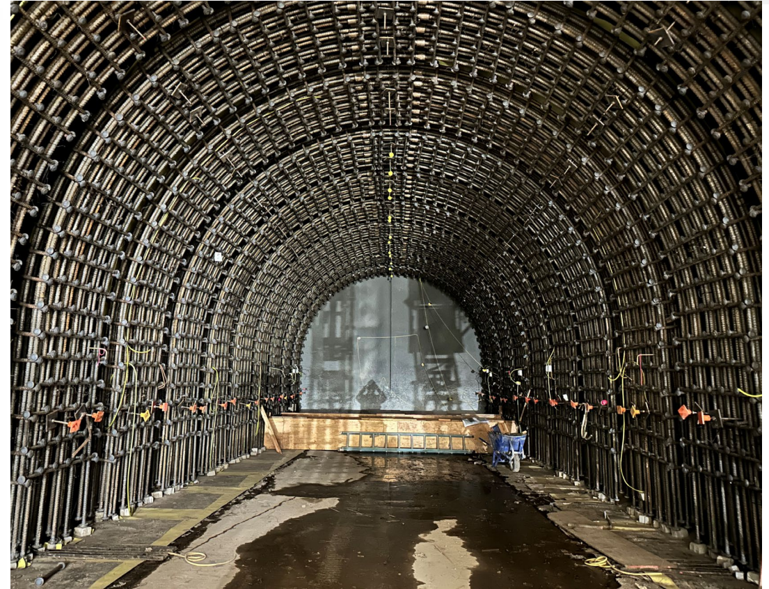
February 2025 Arch reinforcing steel in downstream leg
