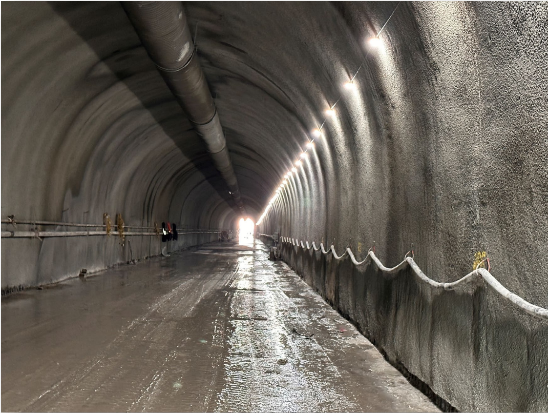
April 2024 Completed tunnel excavation and initial lining
