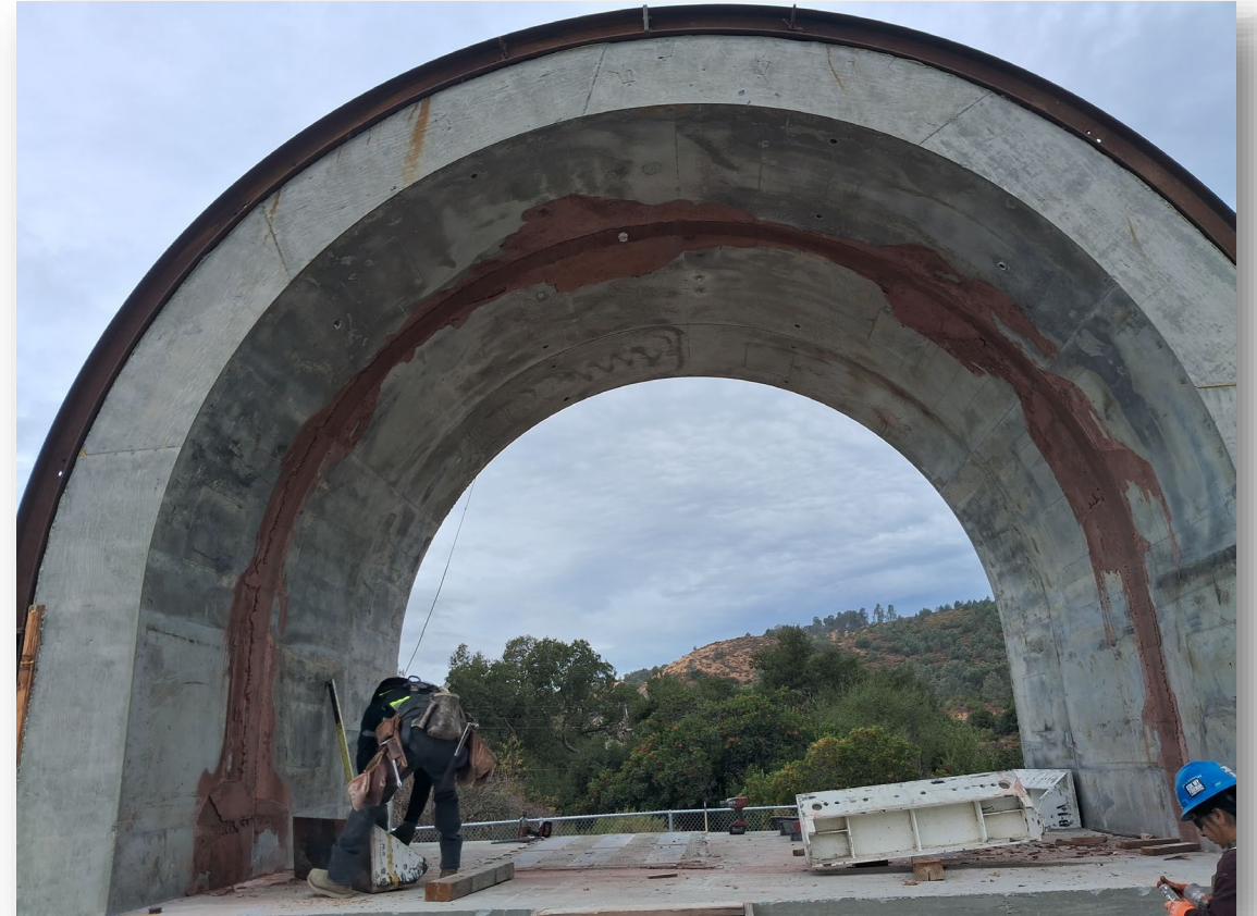
November 2024 Concrete placement completed in the mockup
