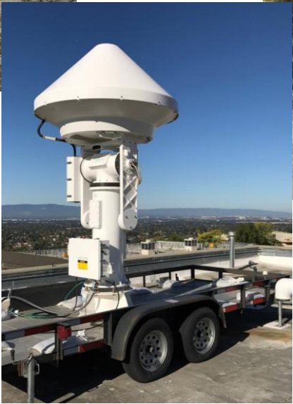
X-band radar on Penitencia Water Treatment Plant rooftop
