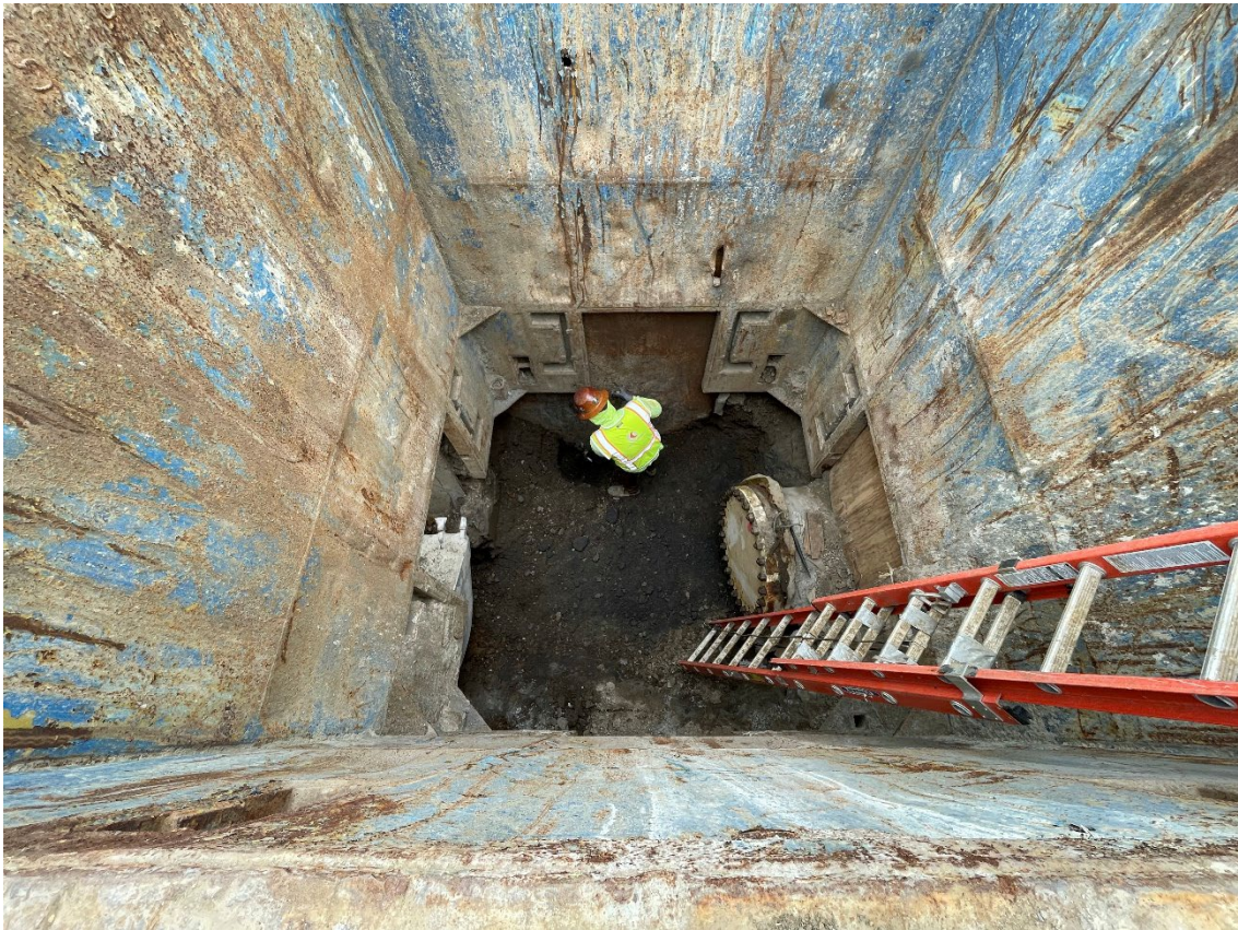
Tie-In Connection to Existing 36" Recycled Water Pipeline
