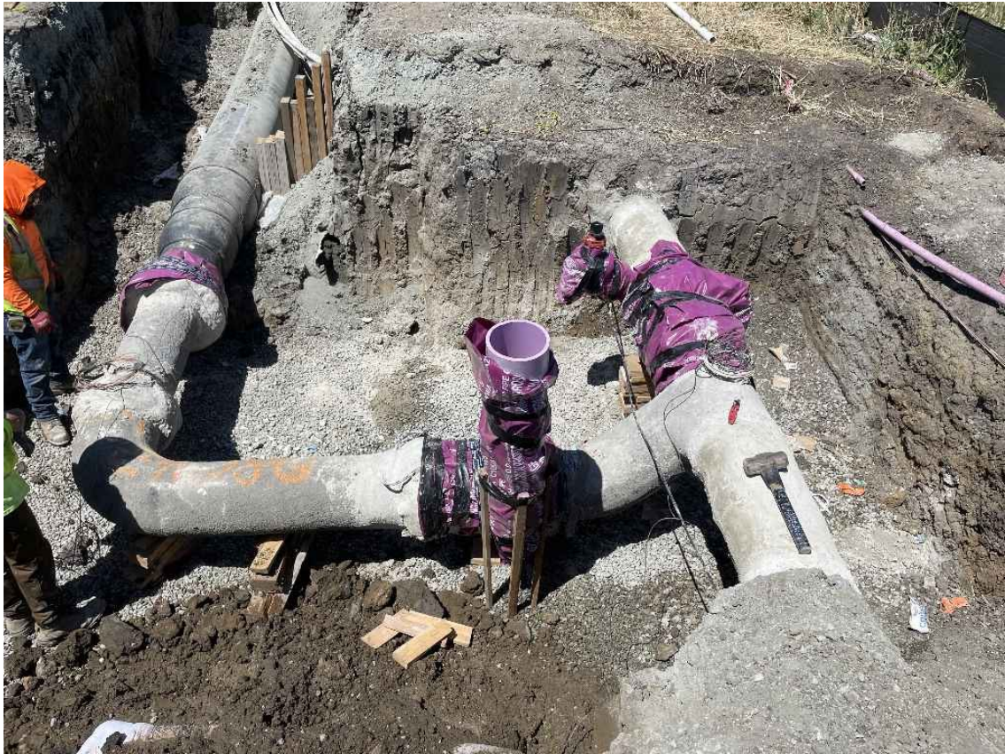
Tie-In Connection to Existing 12" Recycled Water Pipeline
