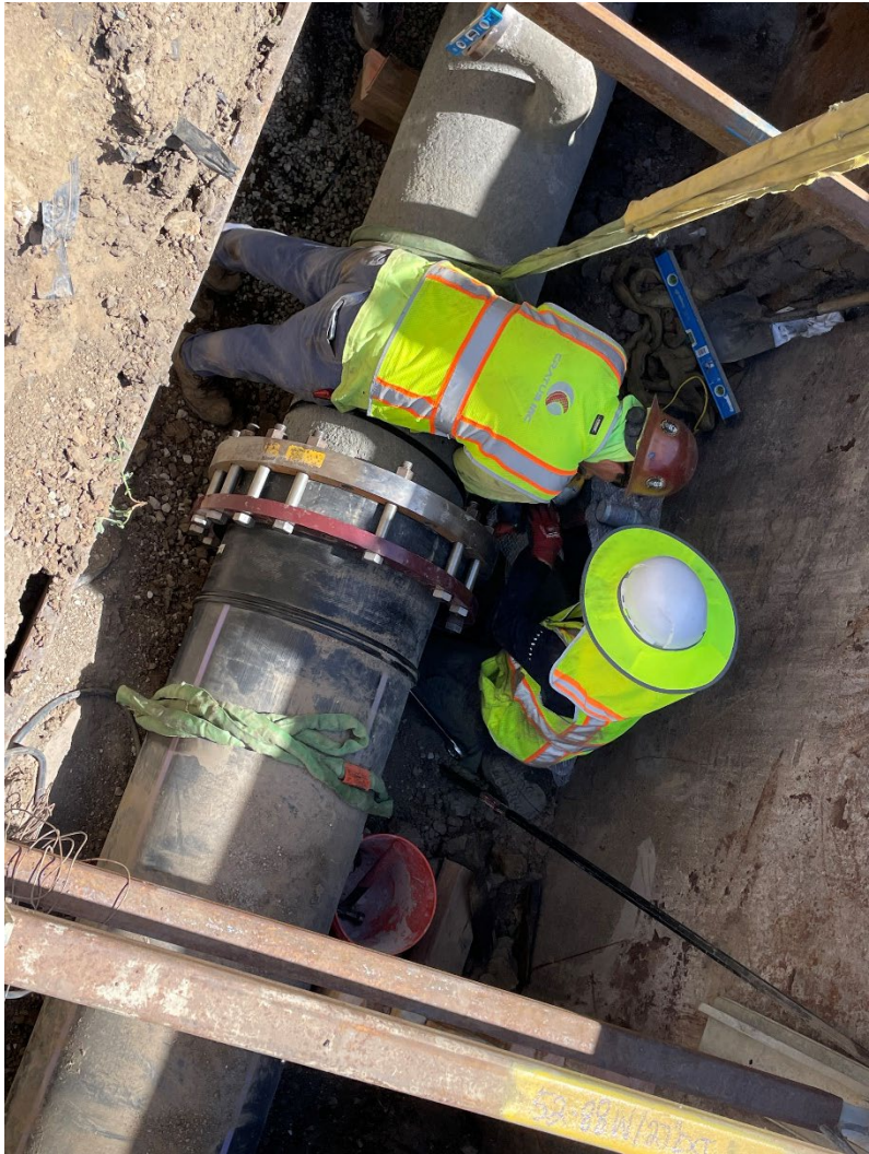
Tie-In Connection to Existing 36" Recycled Water Pipeline
