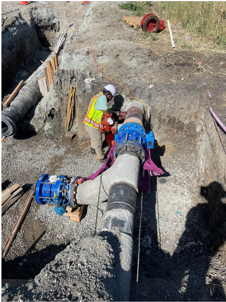
Tie-In Connection to Existing 12" Recycled Water Pipeline
