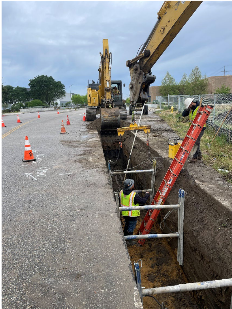
Installation of Shoring System
