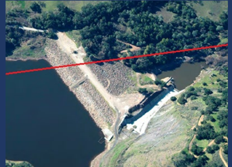
Calaveras Fault crossing embankment
