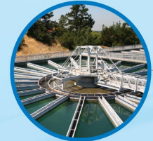
Rinconada Water Treatment Plant
