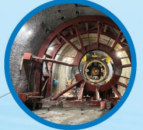
Anderson Dam Tunnel and Seismic Retrofit Projects
