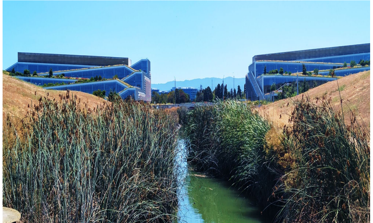
Sunnyvale West Channel, facing south towards Google's Sunnyvale campus
