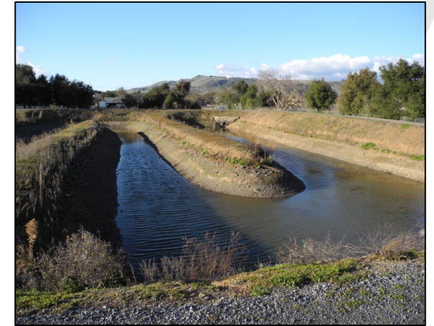
Main Avenue Recharge Ponds
