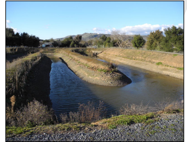
Main Avenue Recharge Ponds
