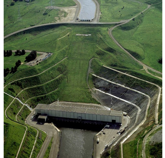
Harvey O. Banks Delta Pumping Plant, California DWR.
