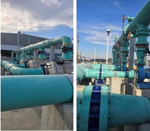
Plant-wide valve replacement project
