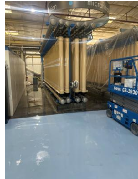
MF membrane replacement
