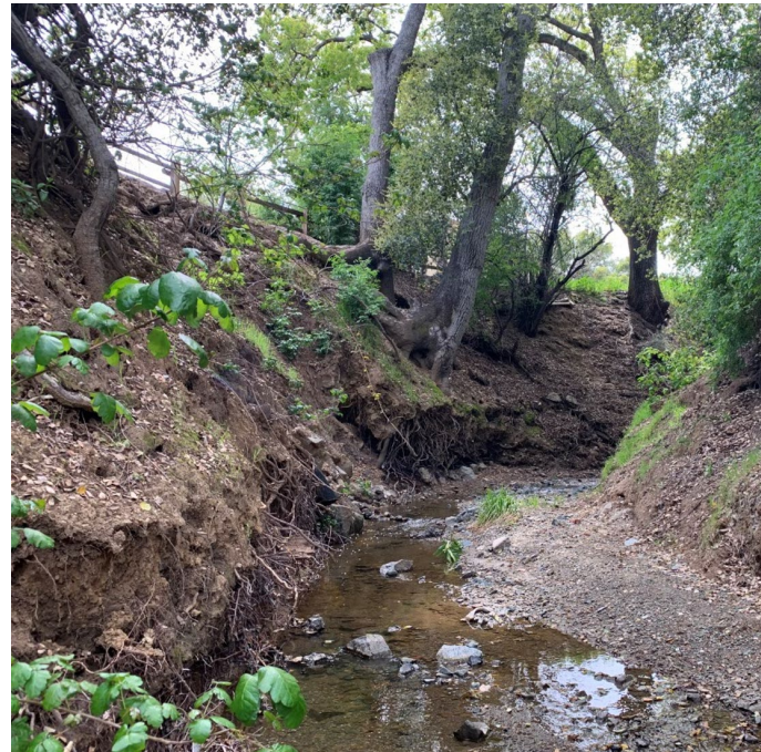
Regnart Creek Rehabilitation Project – F8
