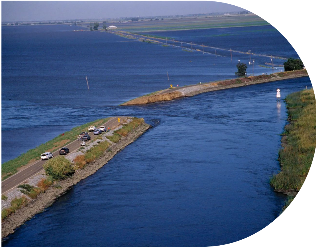
Pictured above: Levee failure at Jones Track during non-flood period
