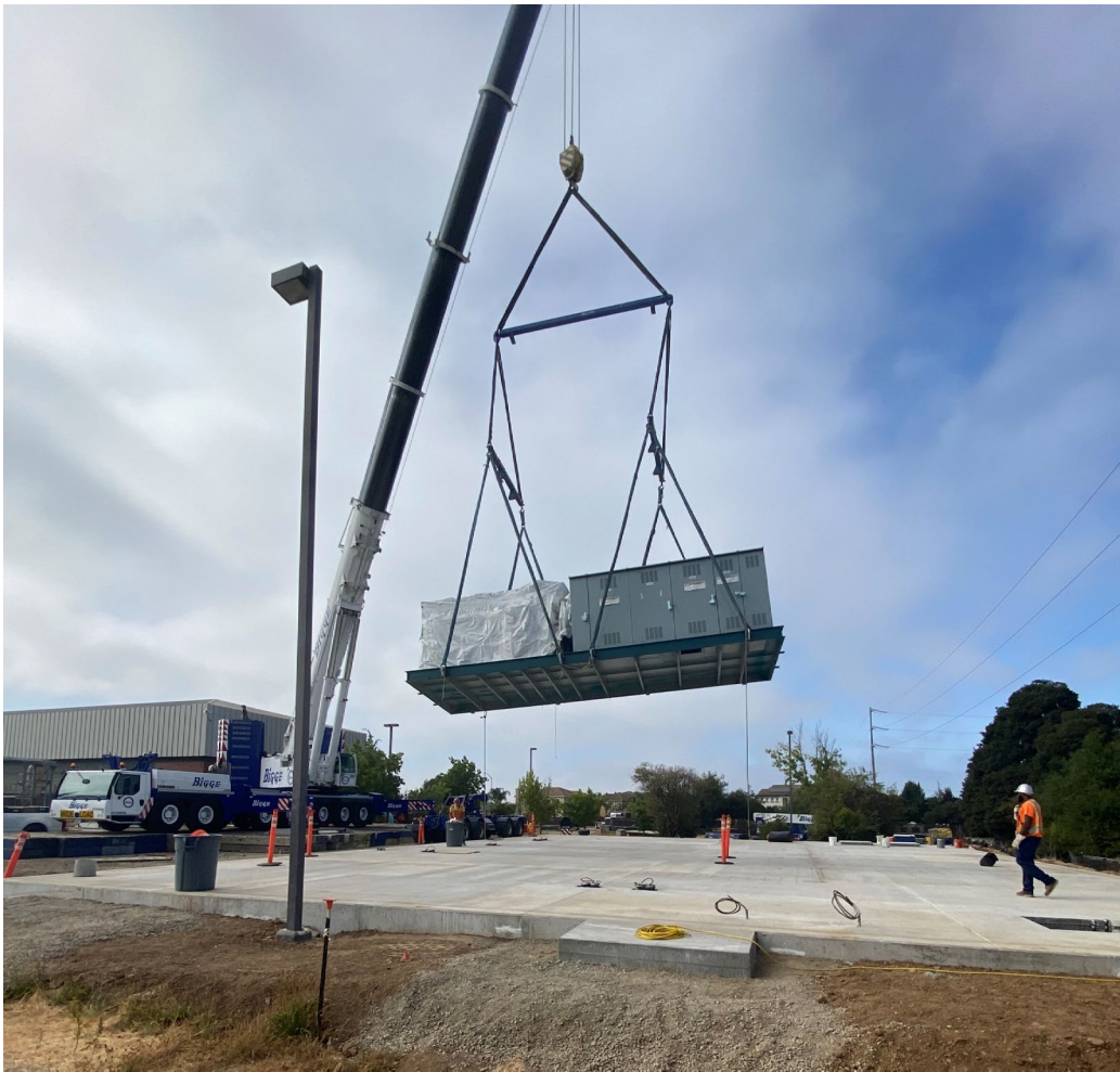
Secondary Unit Substation placed on foundation August 2025
