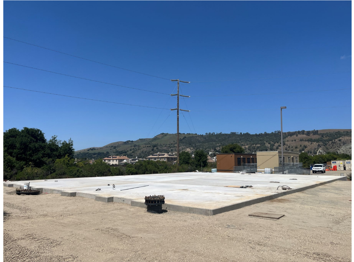
Concrete foundation slab completed in March 2025
