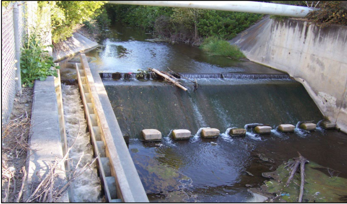
Example of a fish ladder to be modified or reconstructed for improved fish passage
