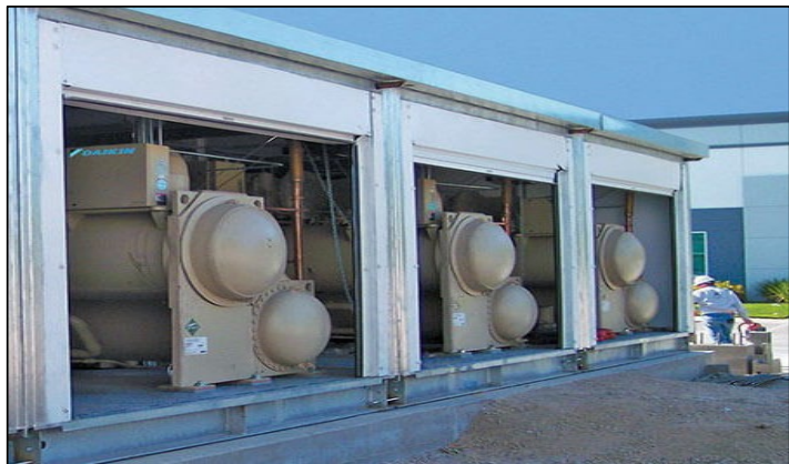
Example of Modular Chiller Plant
