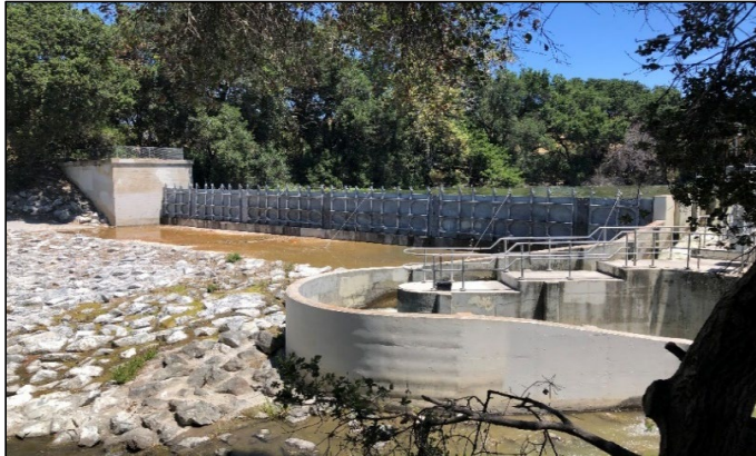
Downstream view of Coyote Percolation Dam, fish ladder, and rock slope protection
