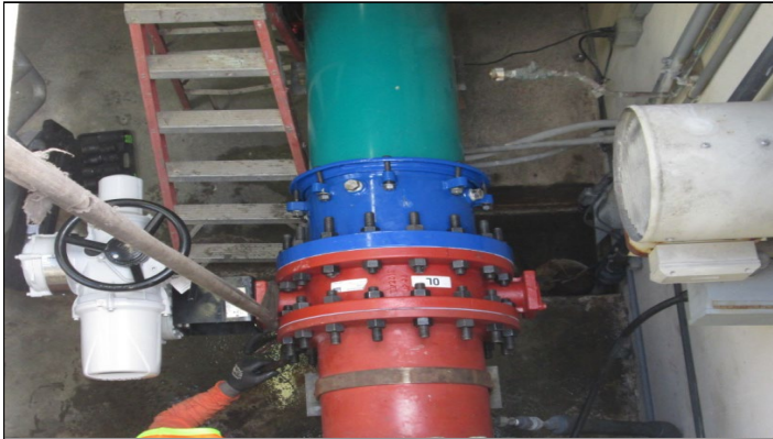
A typical rehabilitated line valve assembly
