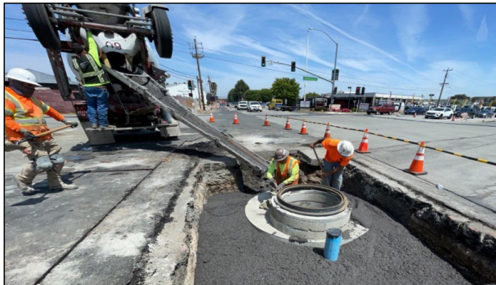
12" RCW turnout connection at the intersection of Monterey Road and Luchessa Ave. in Gilroy, CA
