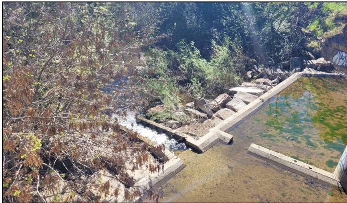
Removal of the Bolsa Road fish barrier allows fish to travel upstream
