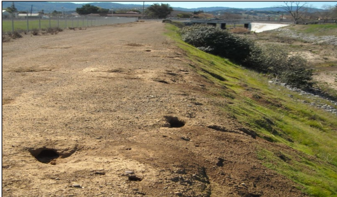
View of damage caused by burrowing animals along West Branch of Llagas Creek in the Uvas/Llagas Watershed
