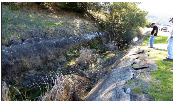
Cracks and separated lining in the canal
