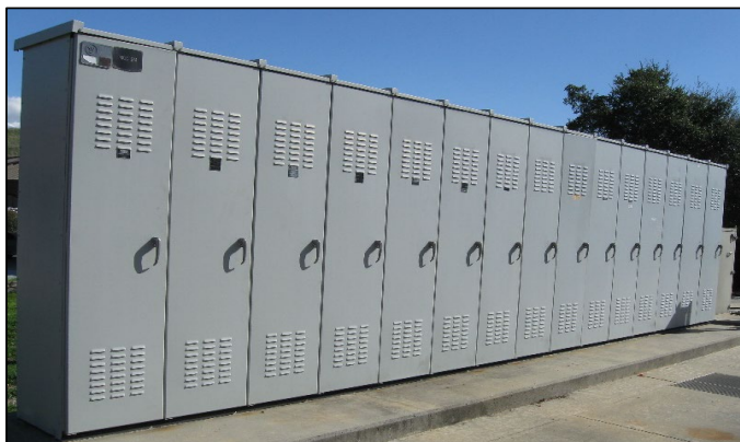
Motor control center switchboard
