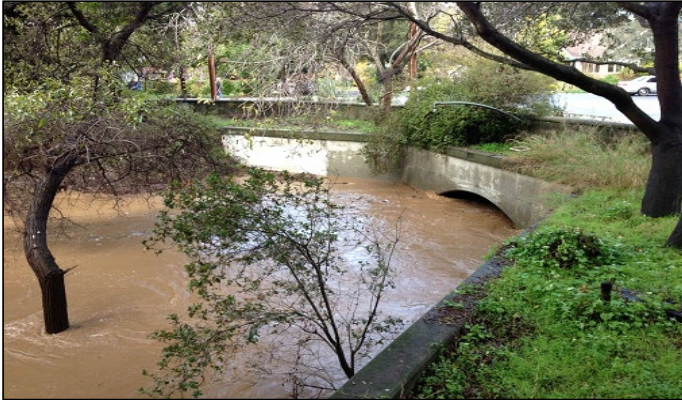
Upstream face of Pope/Chaucer Street with water surface approximately two feet below the soffit
