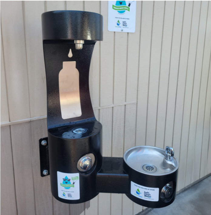
Through a refill station grant, a drinking water fountain was replaced with a dual-function water refill station at Pearl Zanker Elementary School in Milpitas.
