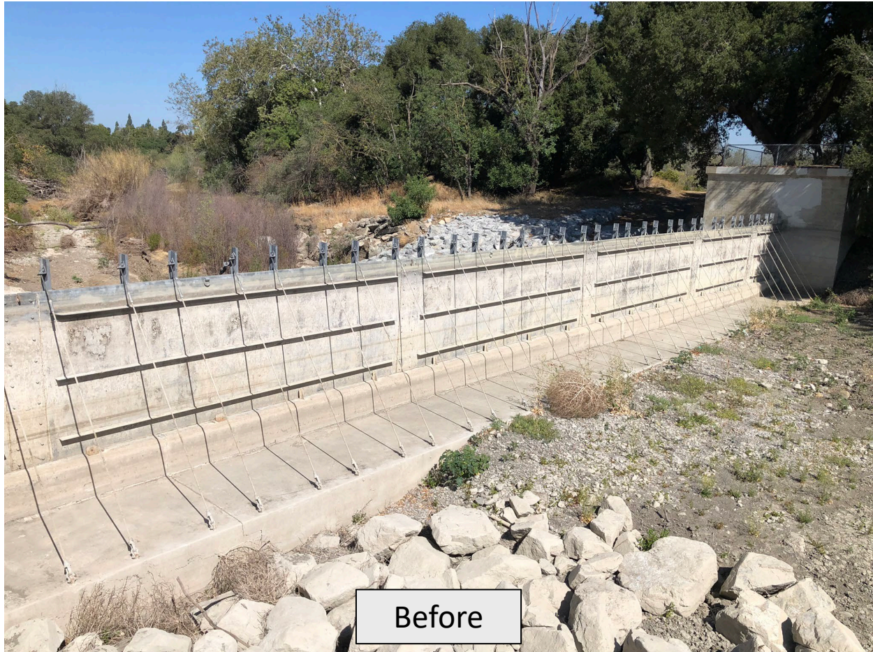
Percolation Dam and Rock Slope Protection
