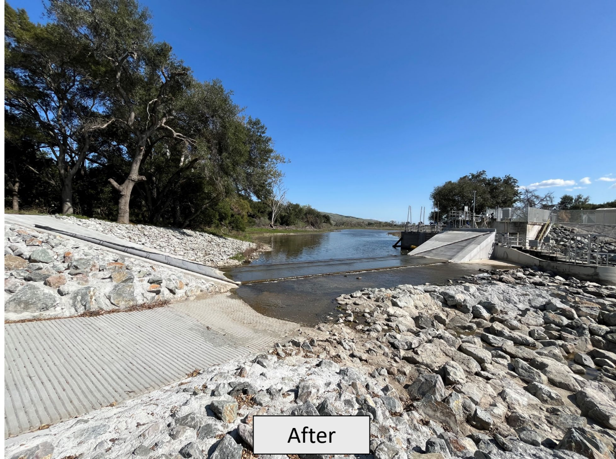
Percolation Dam and Rock Slope Protection
