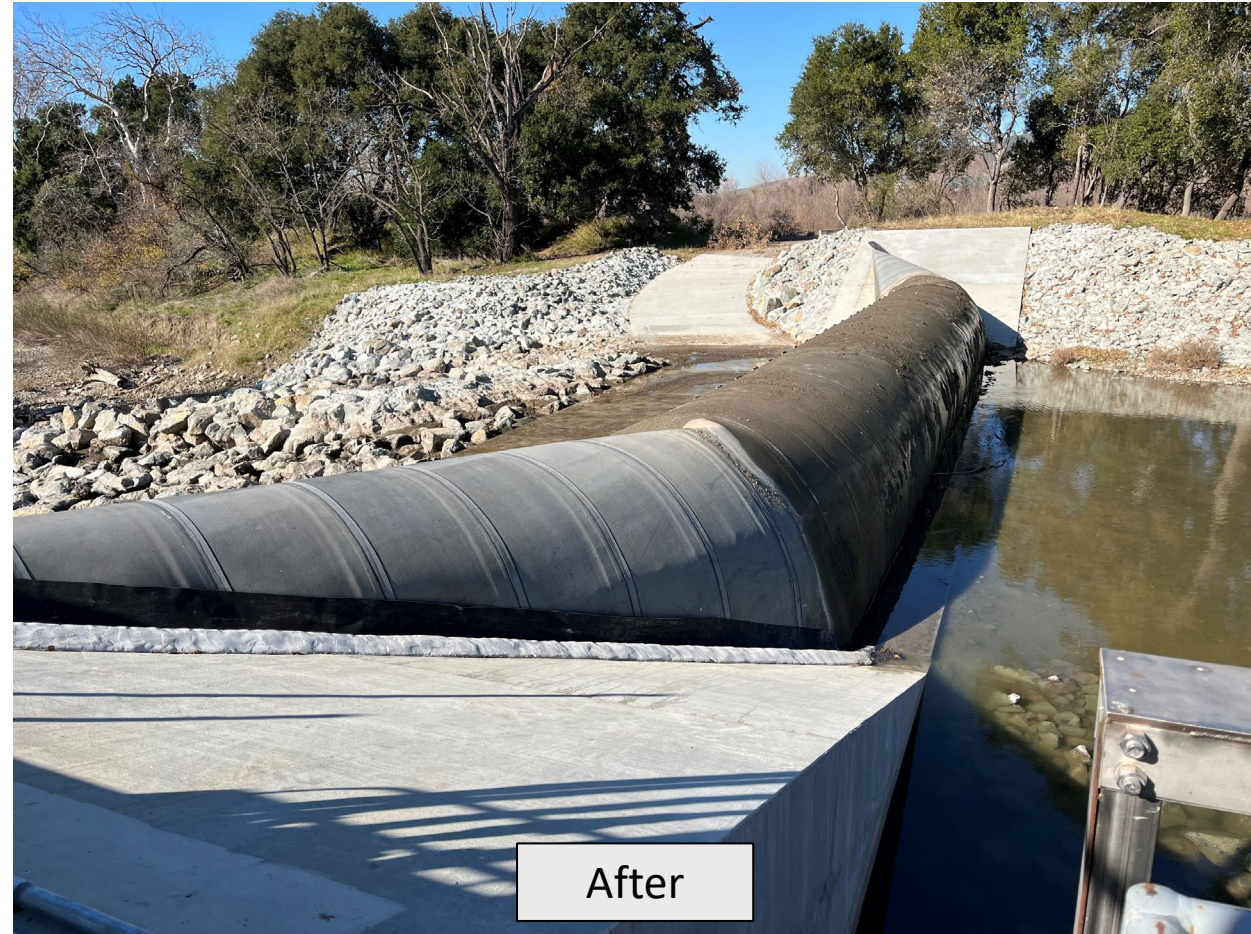
Percolation Dam and Rock Slope Protection
