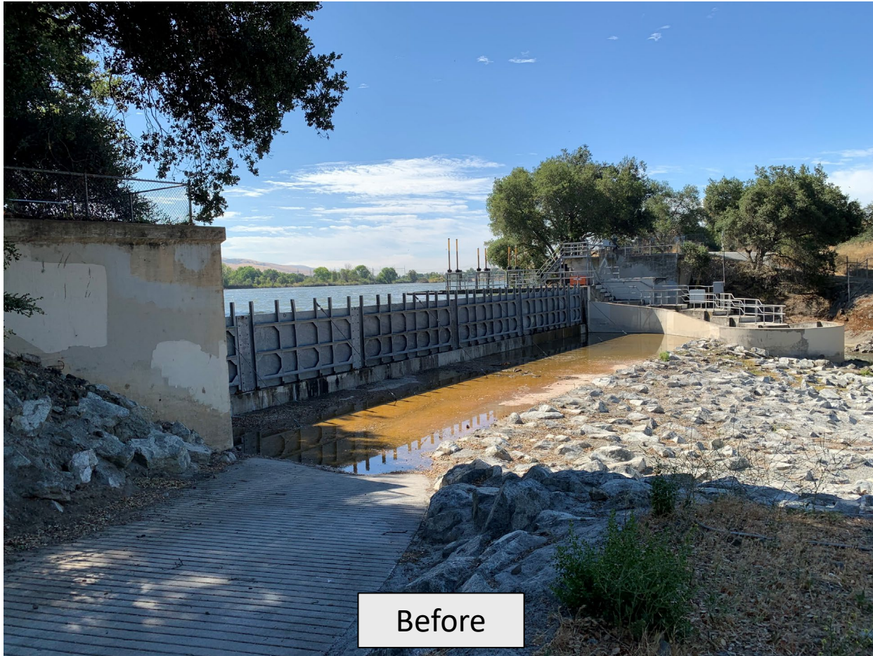
Percolation Dam and Rock Slope Protection
