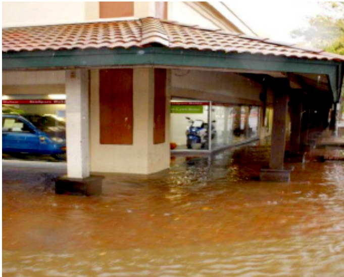
Upper Llagas Creek flooding in Morgan Hill (2009)
