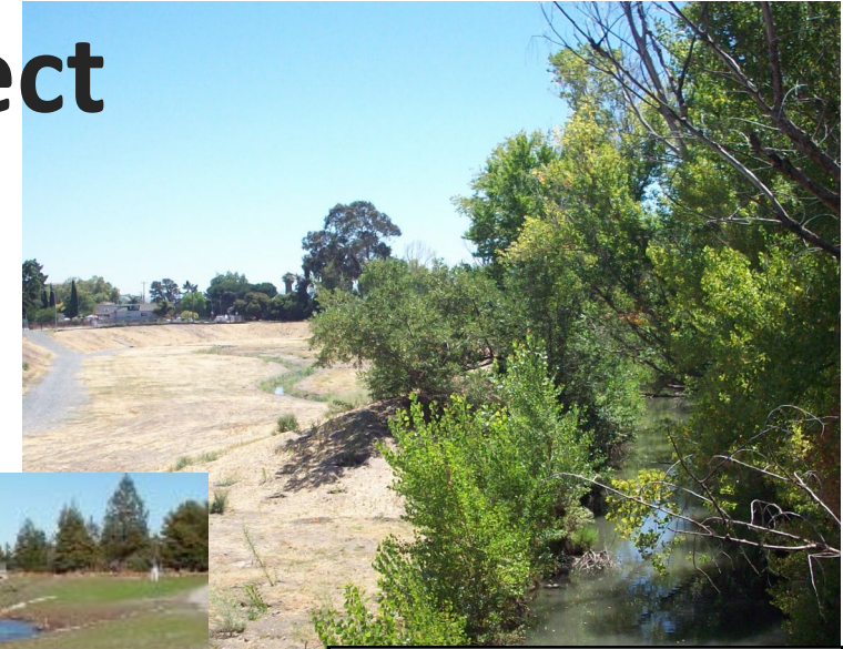
Reach 6 Channel Widening
