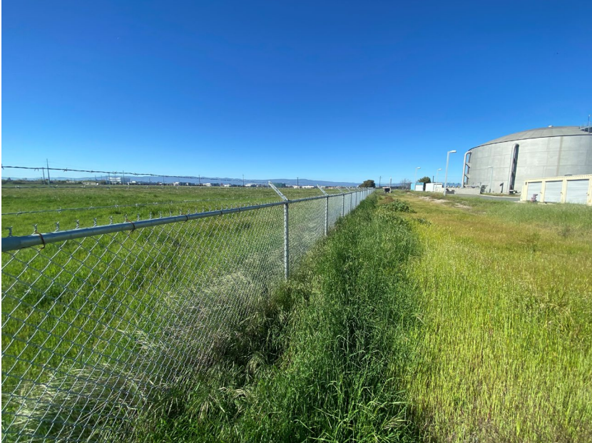
Silicon Valley Advanced Water Purification Center
