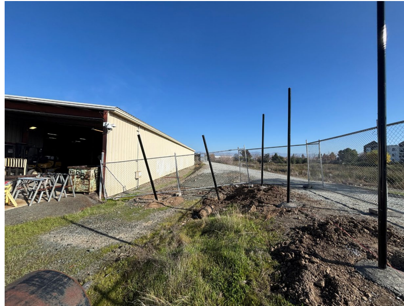
Headquarters Corporate Yard
