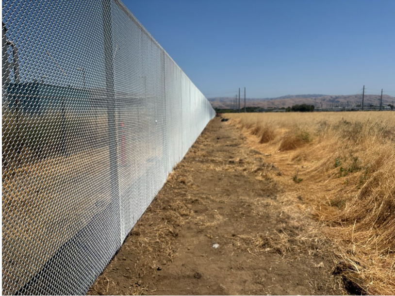
Silicon Valley Advanced Water Purification Center
