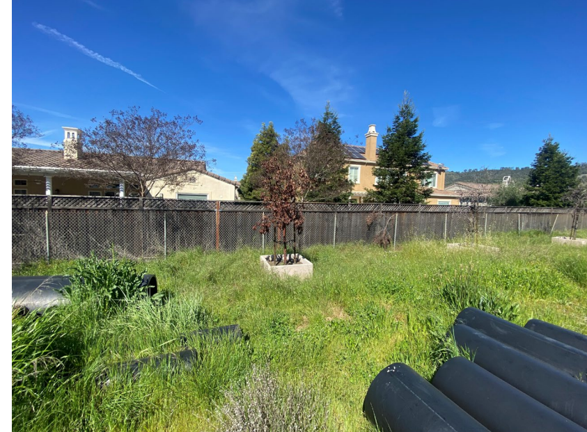
Coyote Pumping Plant
