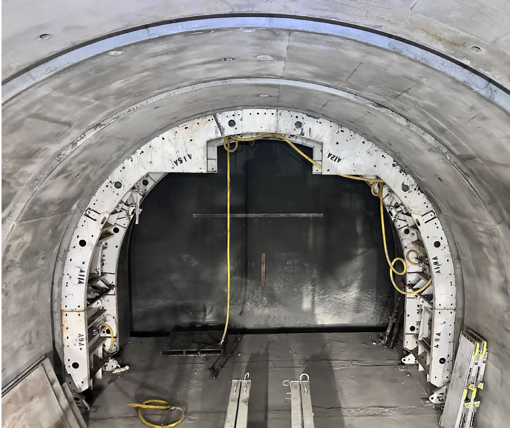
July 2025 – Downstream Leg Invert and arch concrete placed
