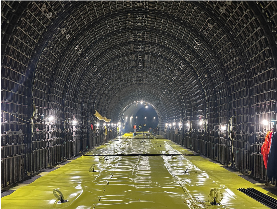
March 2025 – Downstream Leg Arch rebar complete and waterproofing in invert
