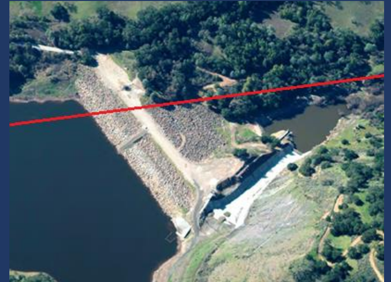
Calaveras Fault crossing embankment
