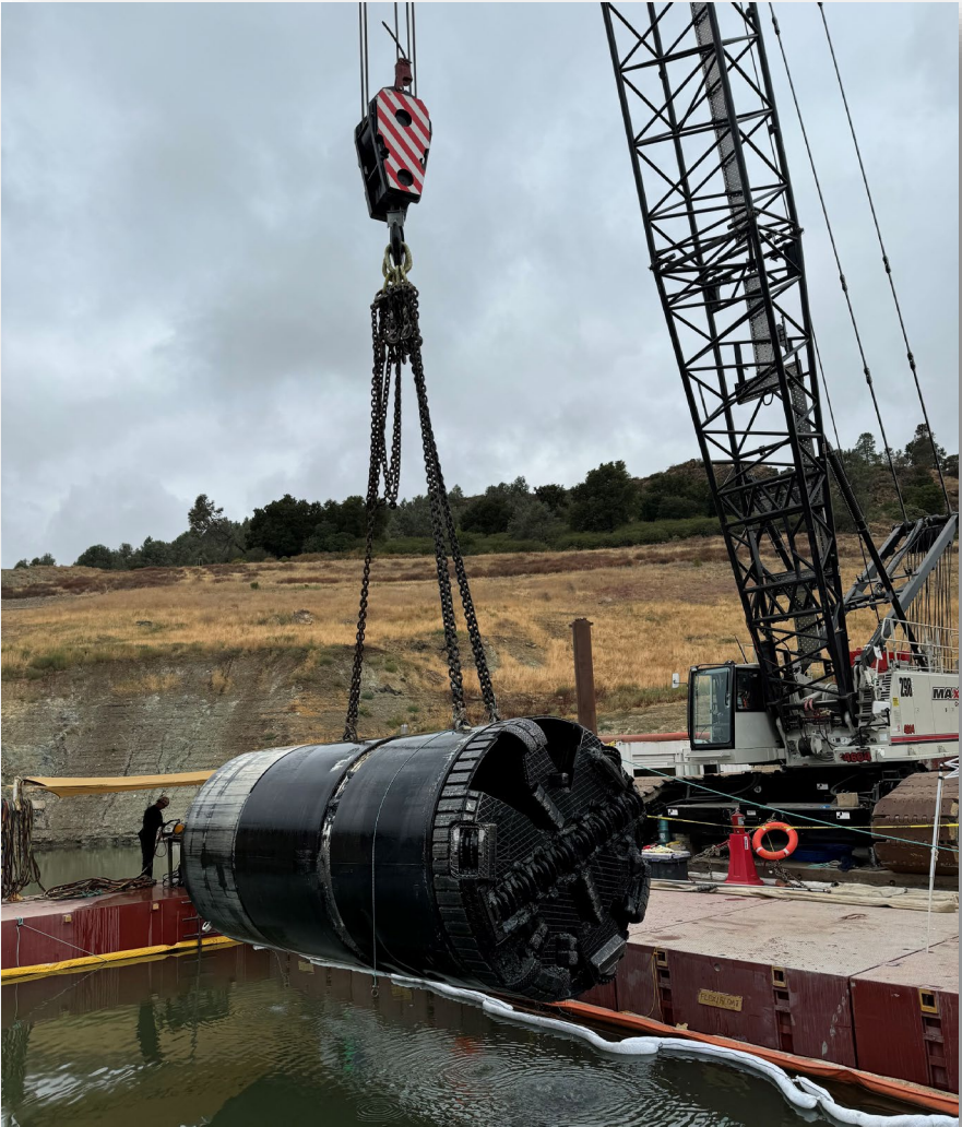
October 2024 – MTBM Retrieval
