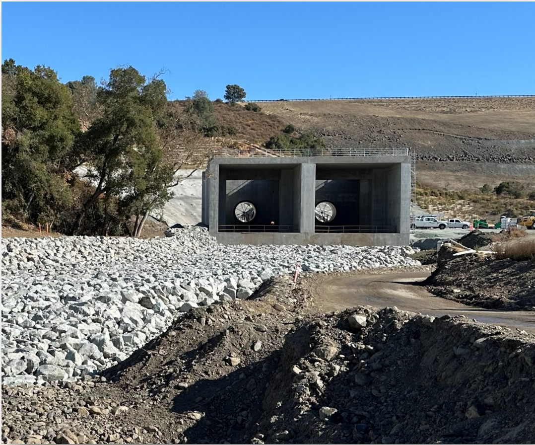
November 2024 – Diversion Outlet Structure
