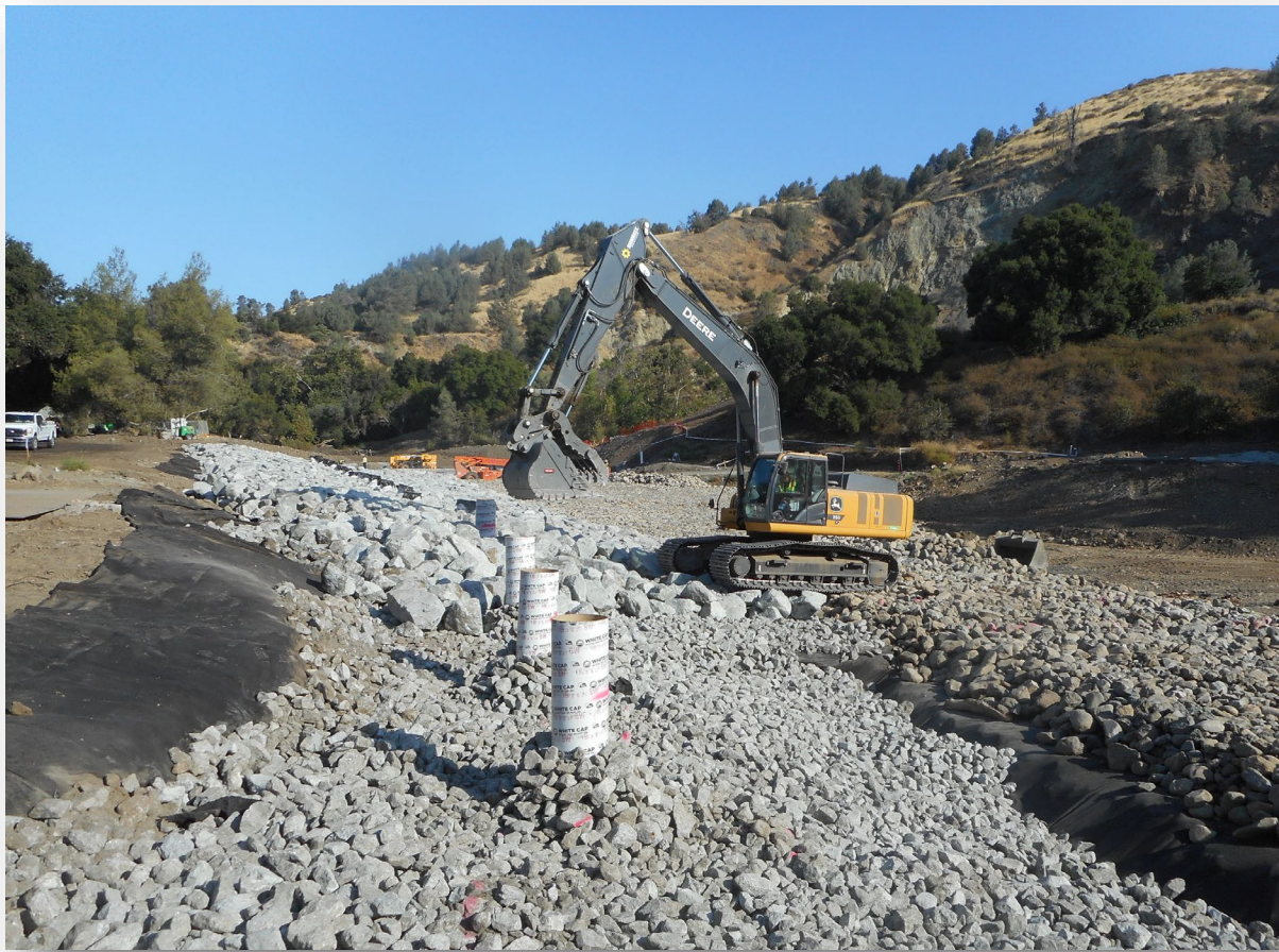
July 2024 – Placing rock in the North Channel
