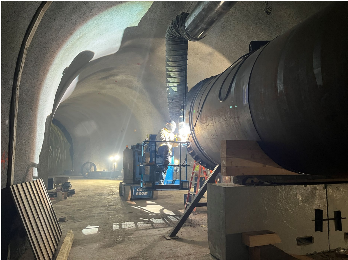
April 2025 Completing the end of the 8-foot diameter MTBM pipe
