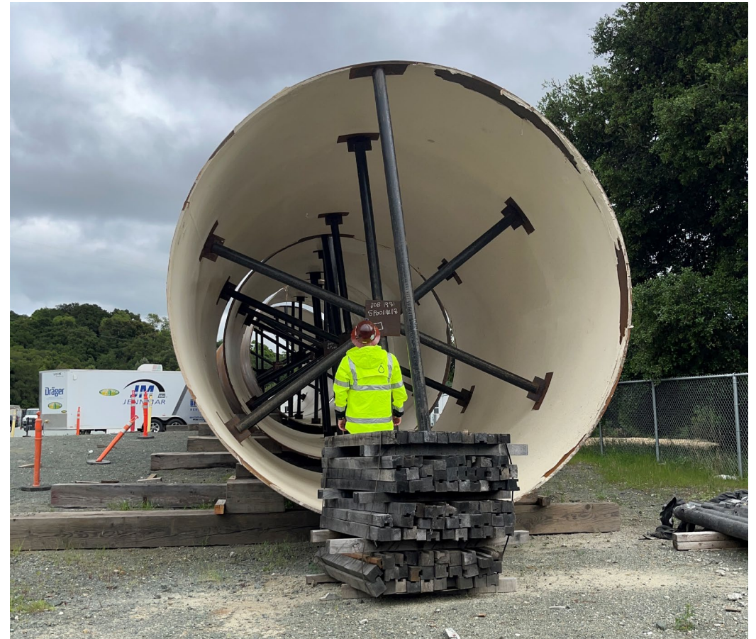
April 2025 Sections of 13-foot diameter steel pipes on site
