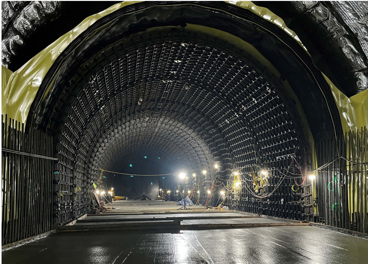
April 2025 – Downstream Leg Invert concrete placed
