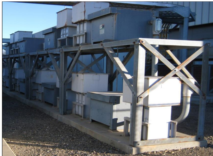
ASD motors at the Coyote Pumping Plant
