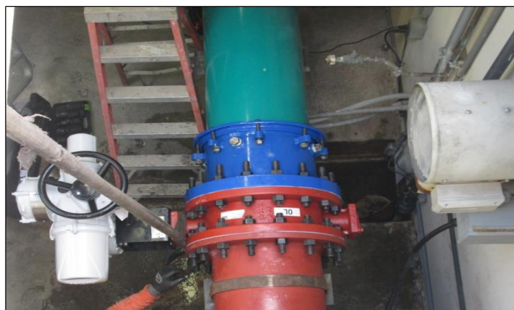
A typical rehabilitated line valve assembly
