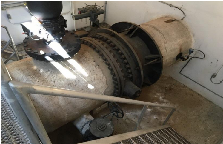
New line valves similar to this will be installed at three locations within the treated water system
