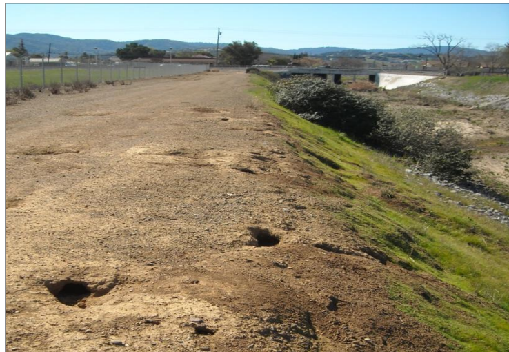
View of damage caused by burrowing animals along West Branch of Llagas Creek in the Uvas/Llagas Watershed
