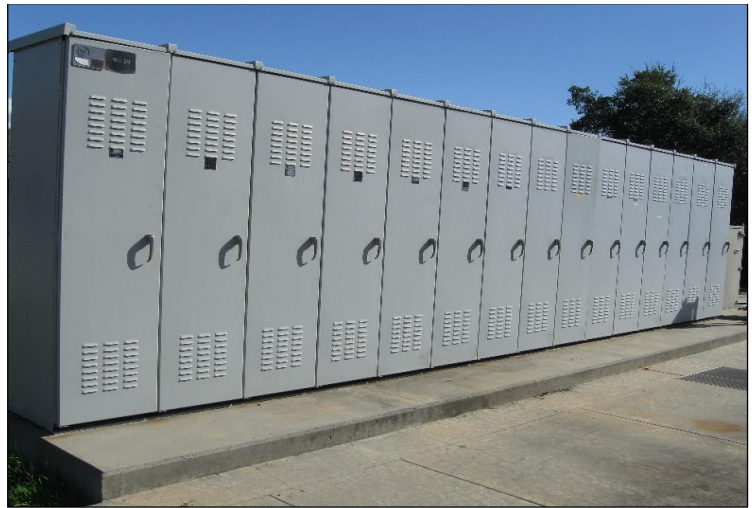
Motor control center switchboard
