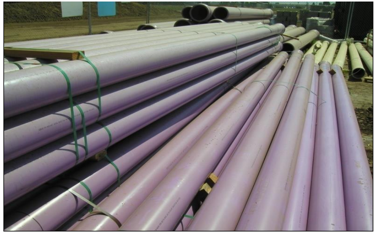
Purple recycled water pipe waiting to be laid during construction of the Immediate Term project
