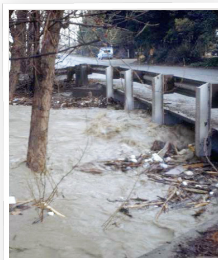
King Road Bridge
