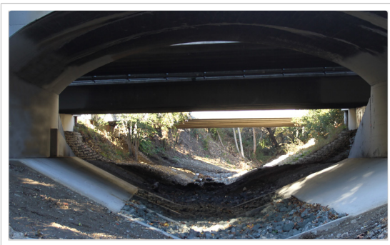
After: Construction of a fish passage channel in Stevens Creek under the bridge face upstream and downstream movements for steelhead trout.
