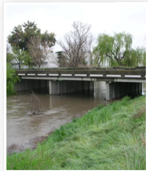
Existing Charcot Road Bridge over Coyote Creek
