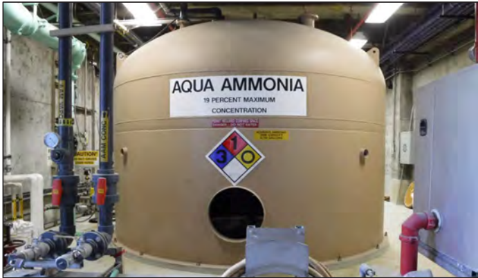
Rinconada Water Treatment Plant Aqua Ammonia Tank
