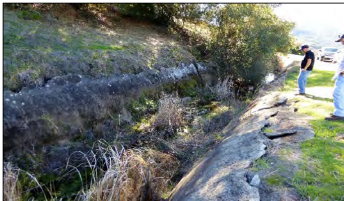
Cracks and separated lining in the canal
