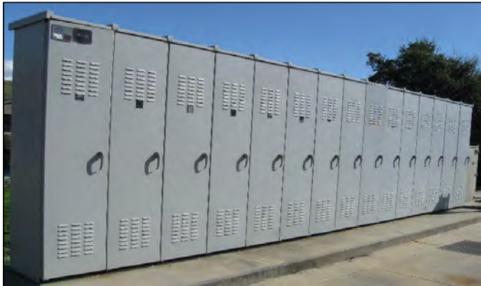
Motor control center switchboard
