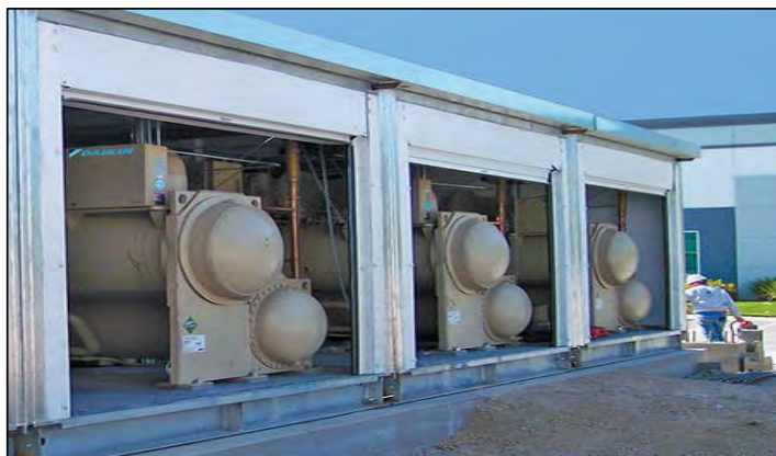
Example of Modular Chiller Plant
