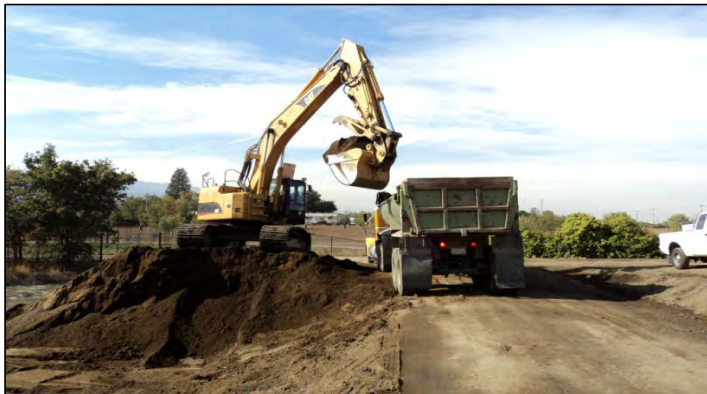
Sludge pond sediment removal at Santa Teresa Water Treatment Plant
