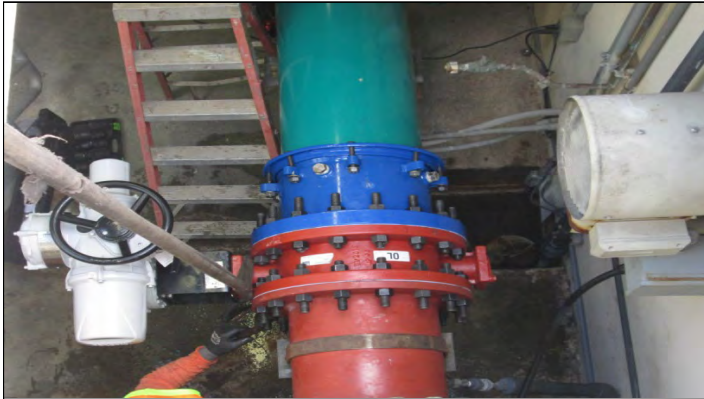
A typical rehabilitated line valve assembly
