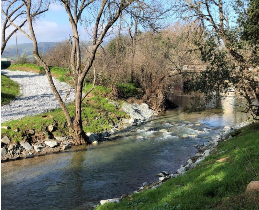
Bolsa Road Fish Passage Improvements
