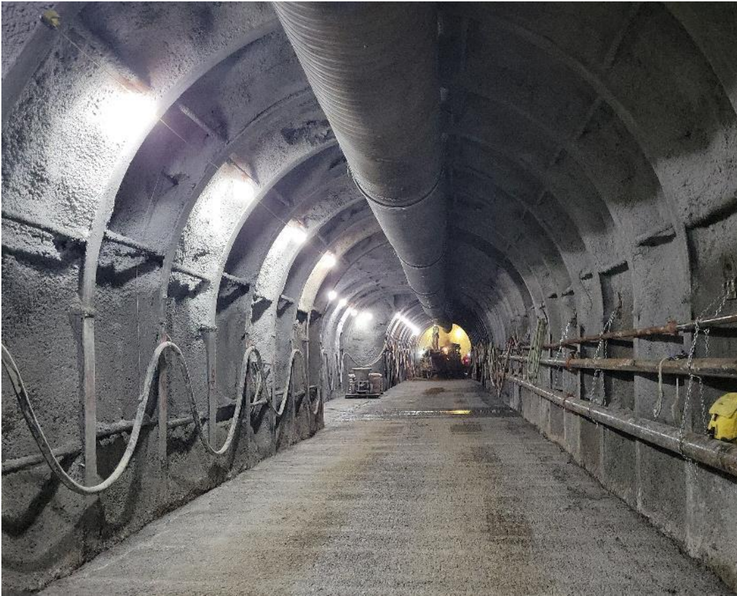
Phase 2A finished tunnel
