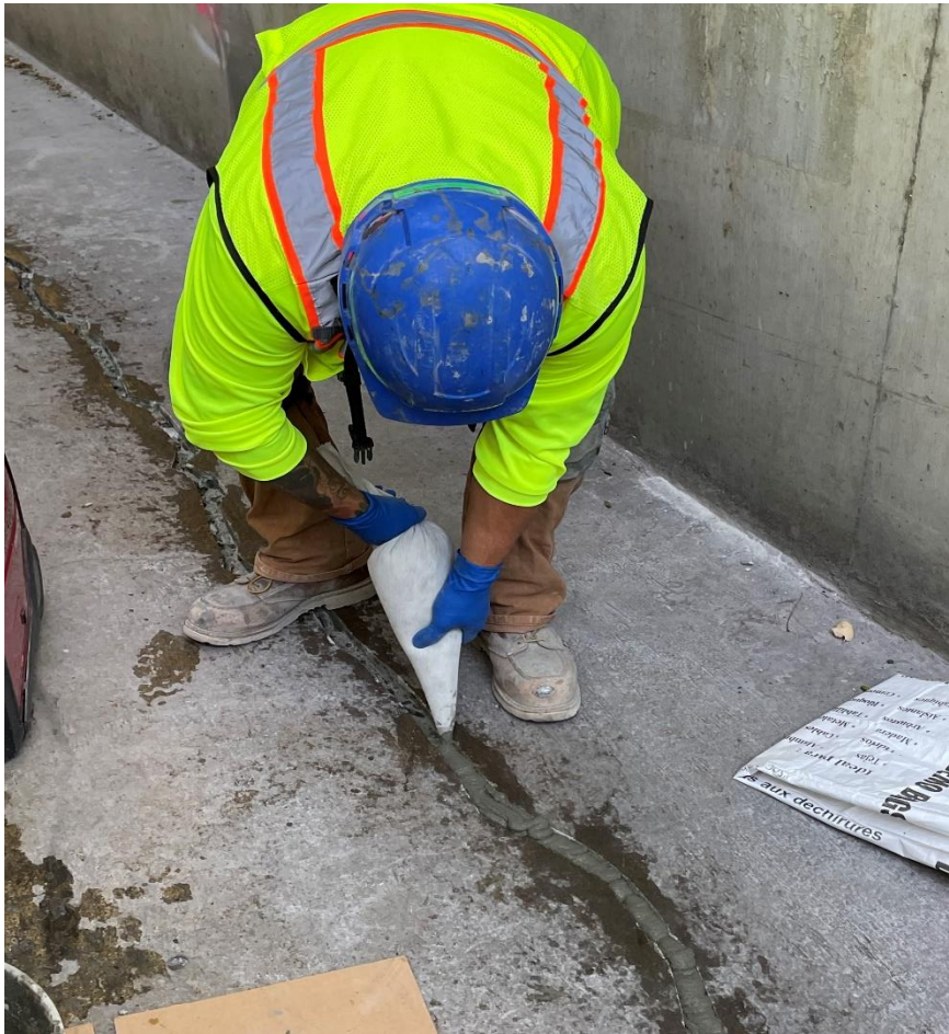
Crack Repair Work on Channel Bottom (During and Post Construction)
