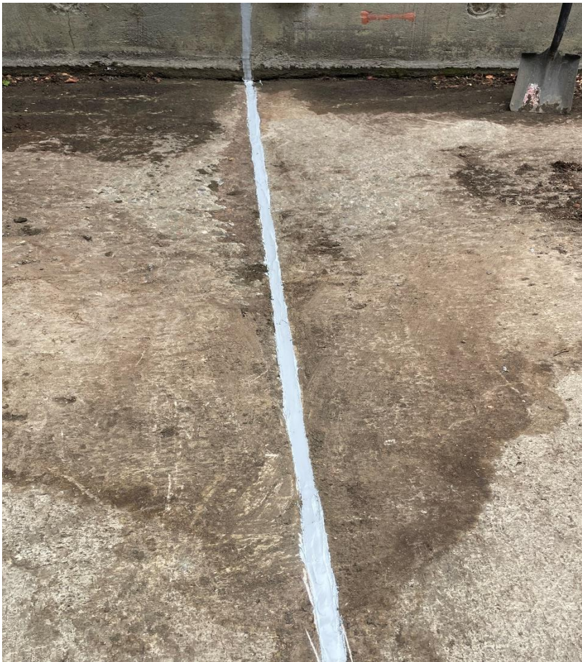
Joint Seal Repair Work (During and Post Construction)
