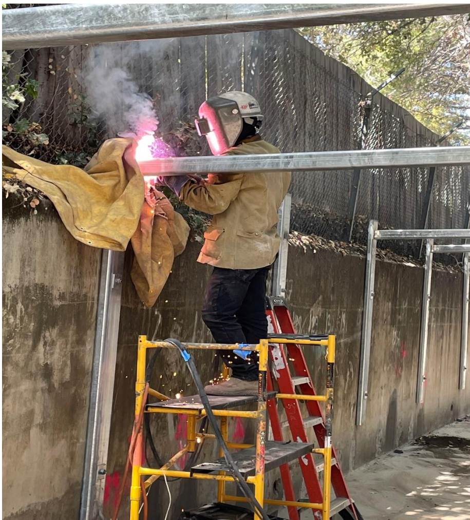
Steel Installation Work at Hale Creek
