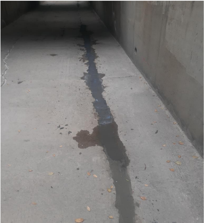
Crack Repair Work on Channel Bottom (During and Post Construction)
