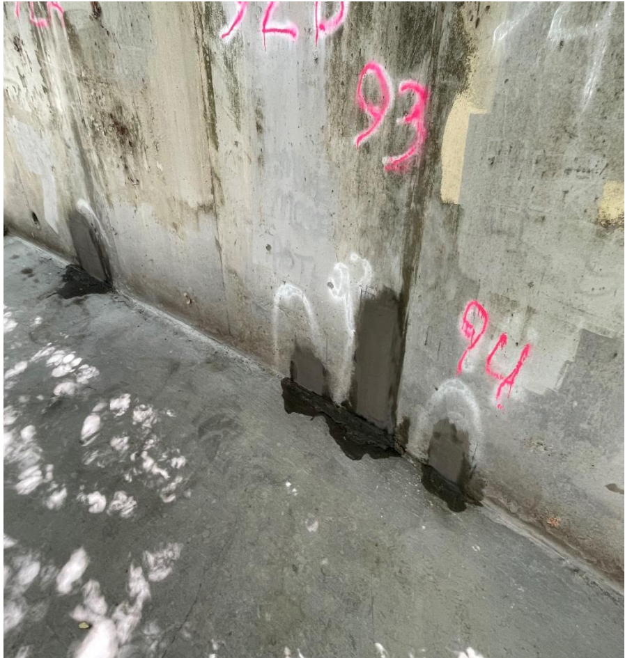
Wall Spall Repair Work (During and Post Construction)
