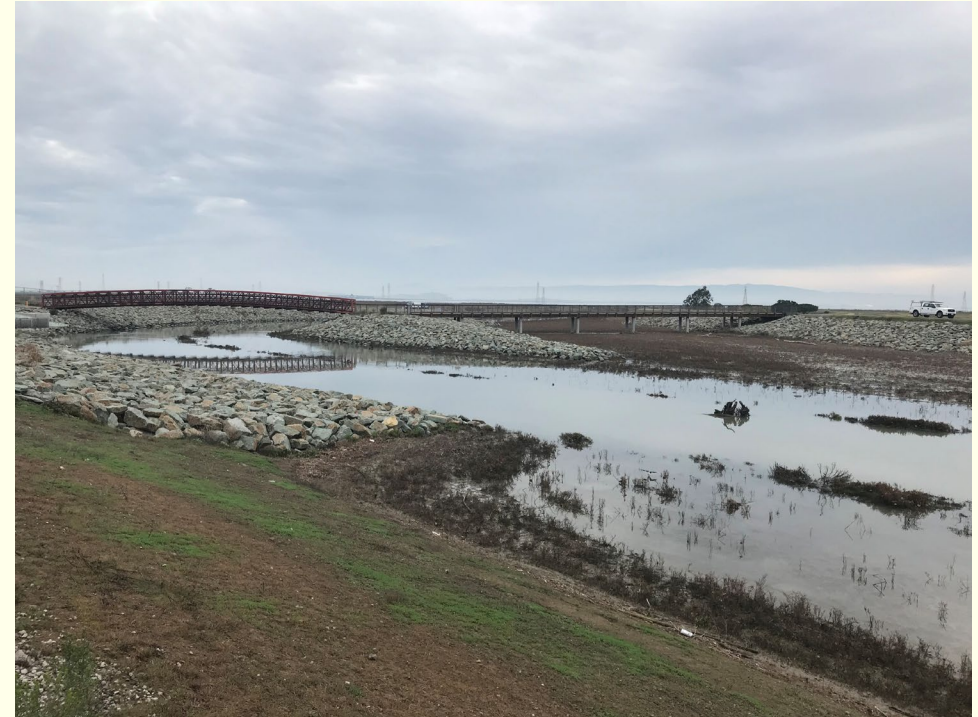
Completed Reach 1 Project at Friendship Bridge
