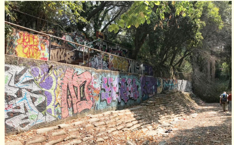
Concrete terrace at Site 2
