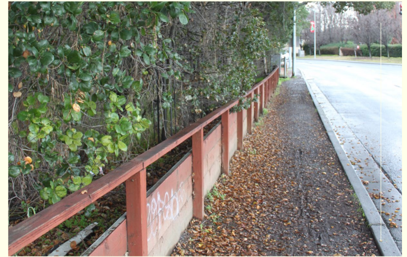
Temporary wooden parapet at University Ave
