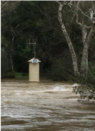
Madrone stream gauge at Coyote Creek
