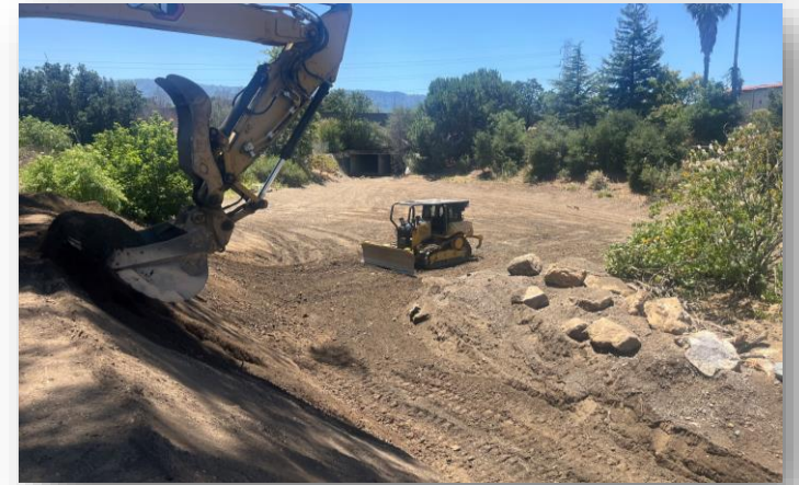
San Tomas Aquino Creek – U/S Westmont Ave (San Jose)
