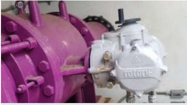
Plunger Valve at Main Avenue Ponds Vault.
