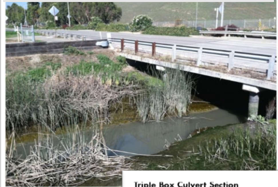
Triple Box Culvert Section
