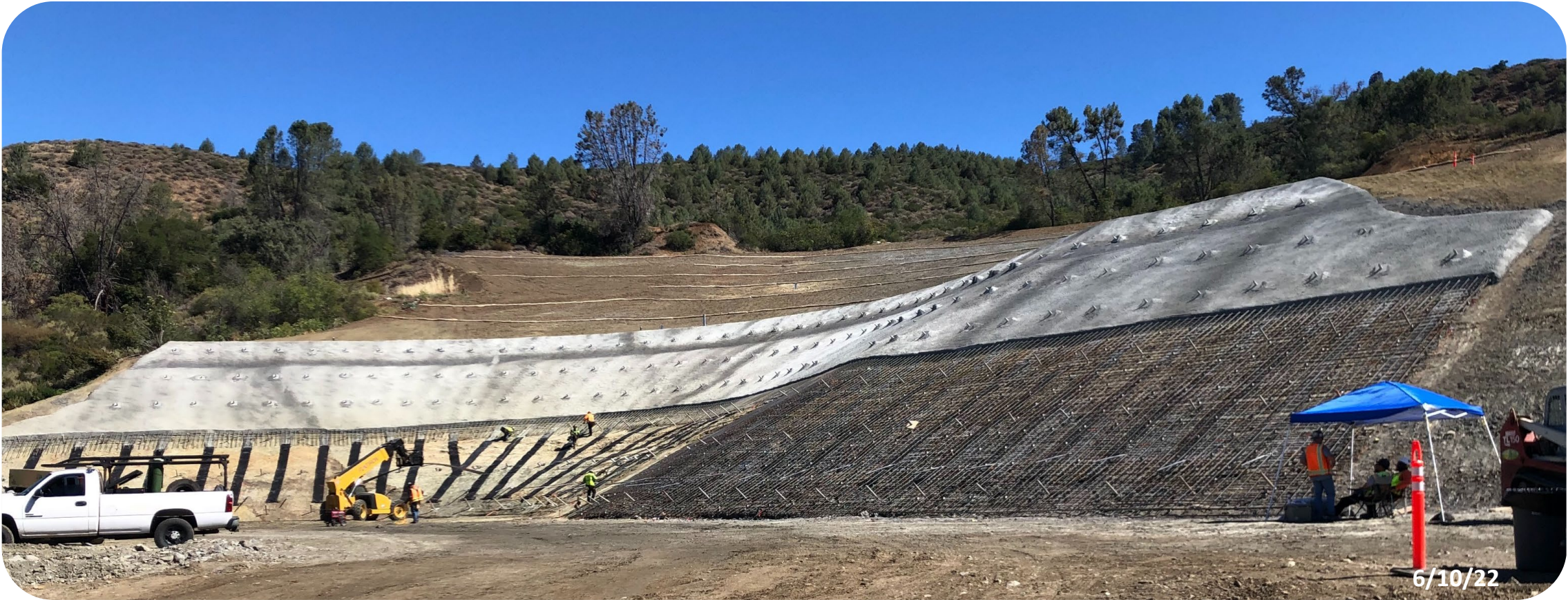
soil nail wall bottom = 300 linear feet
