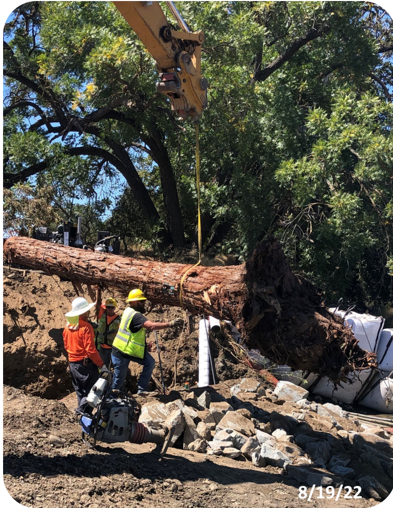
Root wad placement at outfall
