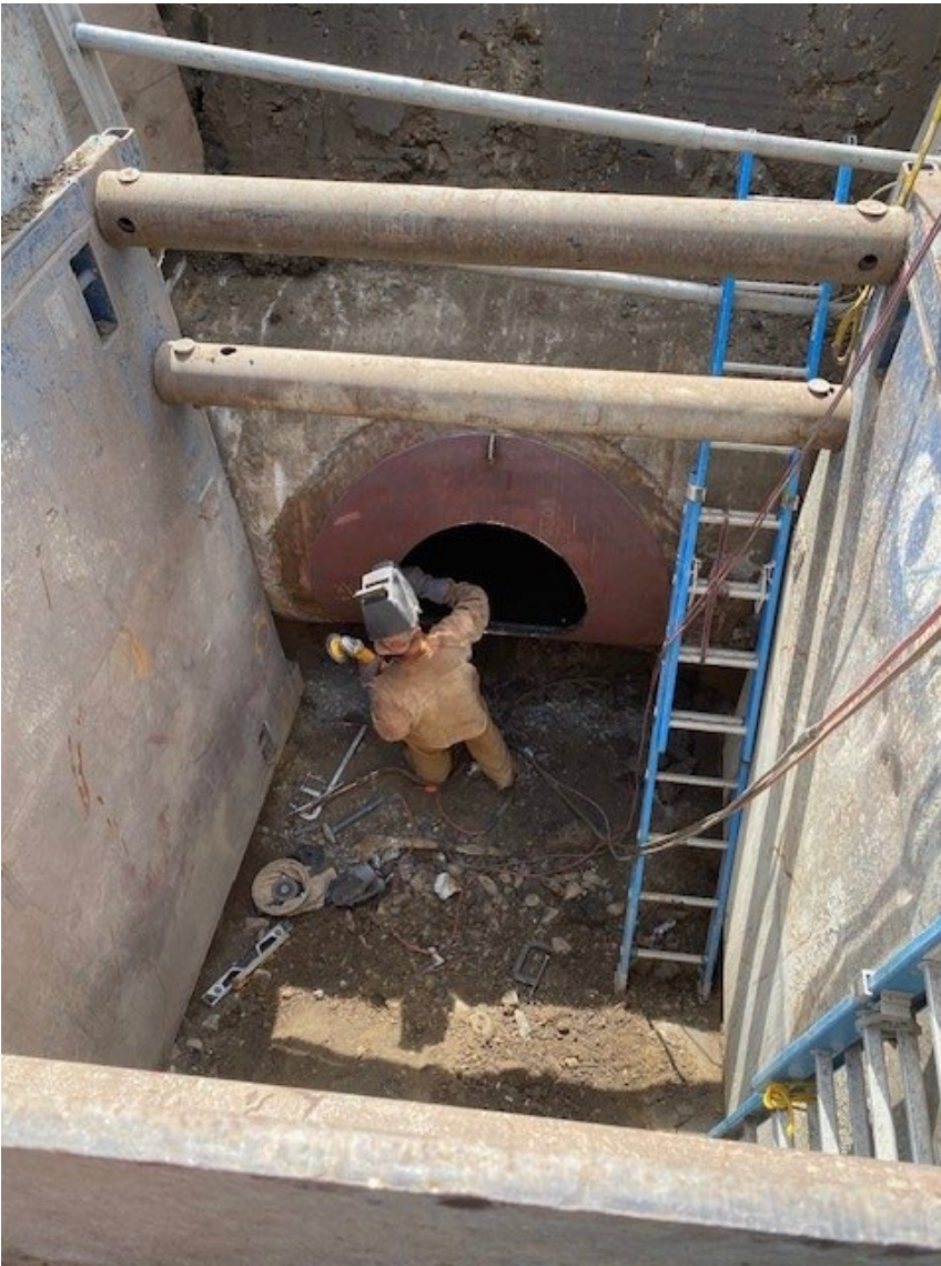
New 36" Cross Valley Pipeline Tie-In to 78" Cross Valley Pipeline
