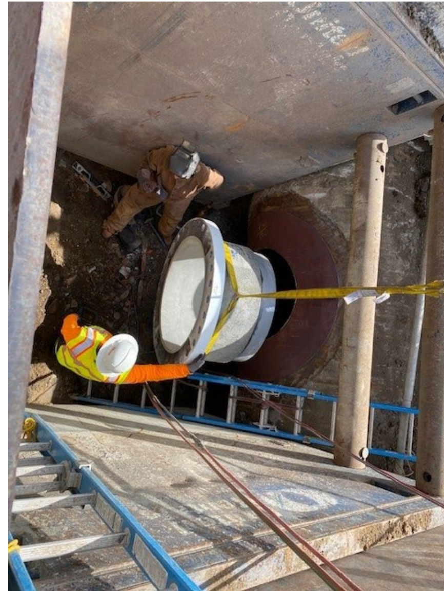
New 36" Cross Valley Pipeline Tie-In to 78" Cross Valley Pipeline
