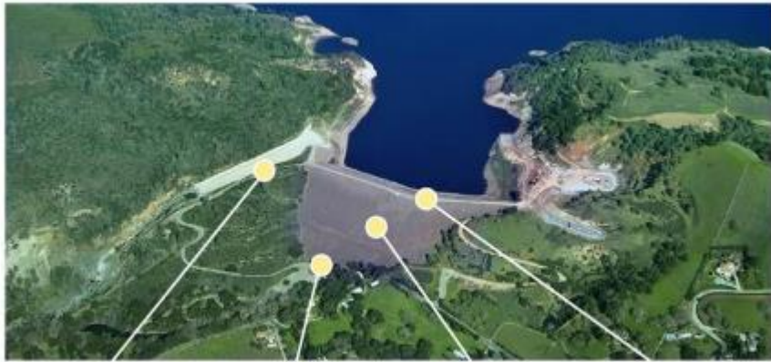
Spillway Outlet pipe Dam embankment Crest of dam
