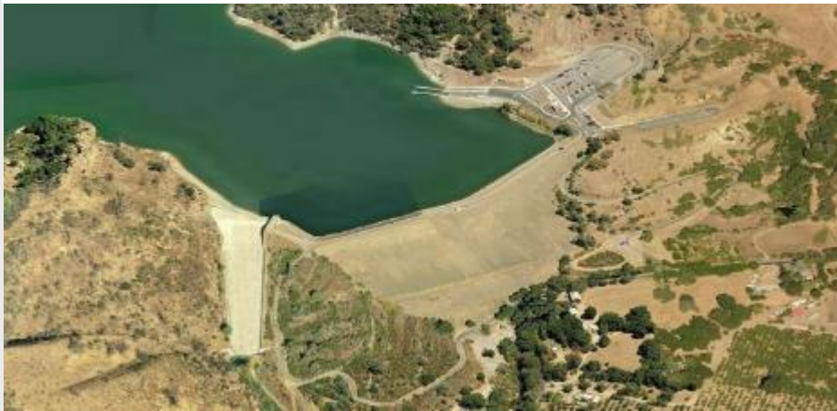
Spillway Outlet pipe Dam embankment Crest of dam
