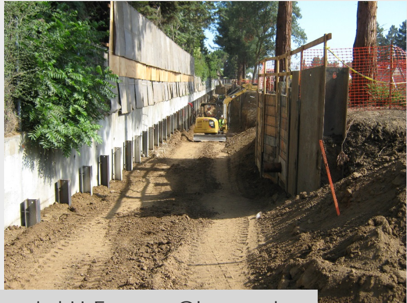
Permanente Creek Special U-Frame Channel
