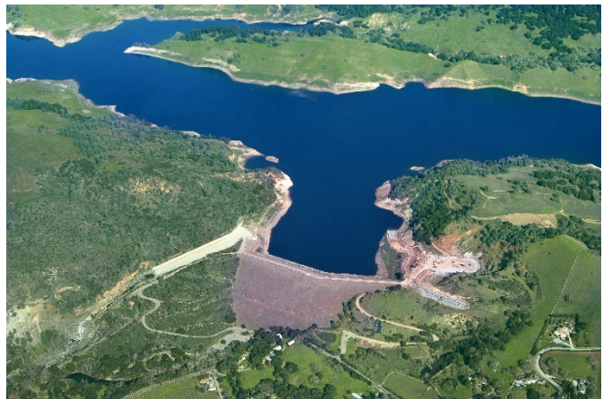
Anderson Reservoir is currently being operated at a reduced capacity due to seismic concerns with the dam at full capacity.
