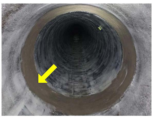
Epoxy mortar covering termination ring
