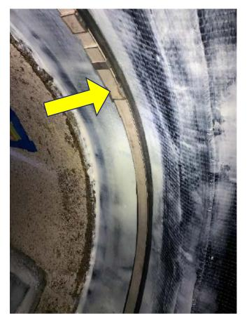
Termination ring at joint of repaired pipe
