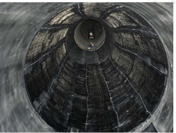
Hoop and Longitudinal Layer of Carbon Fiber
