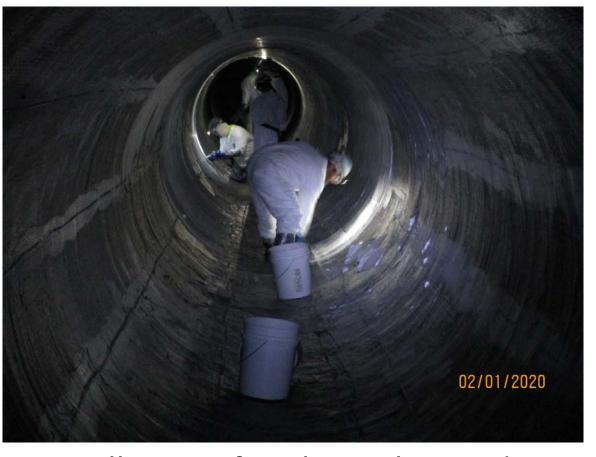
Installation of Carbon Fiber and Thickened Epoxy
