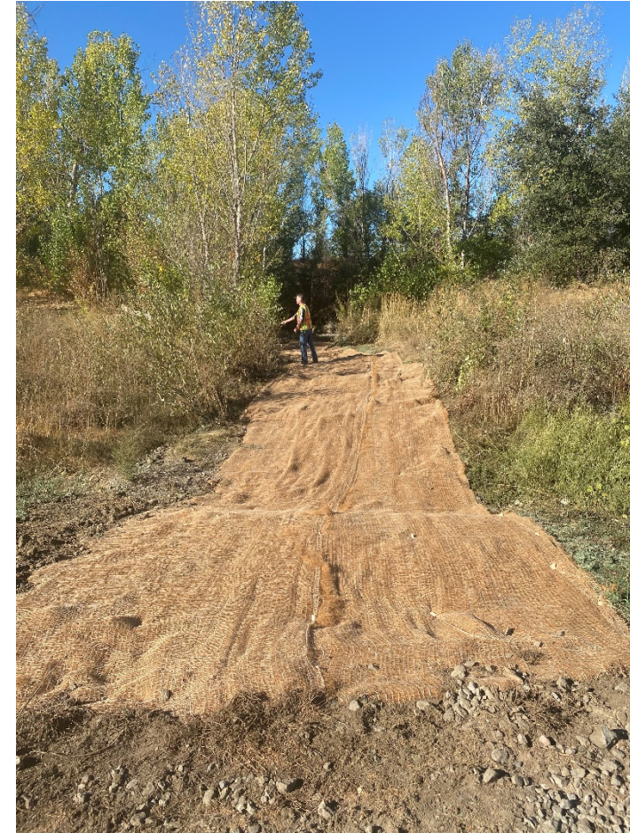
Access Road at Site #2 before and after w/hydroseed and erosion control mat
