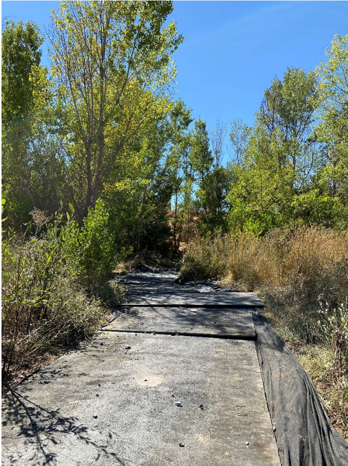
Access Road at Site #2 before and after w/hydroseed and erosion control mat
