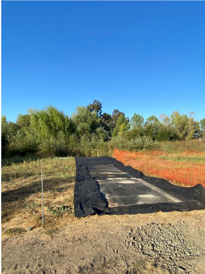
Access Road at Site #1 before and after w/hydroseed and erosion control mat
