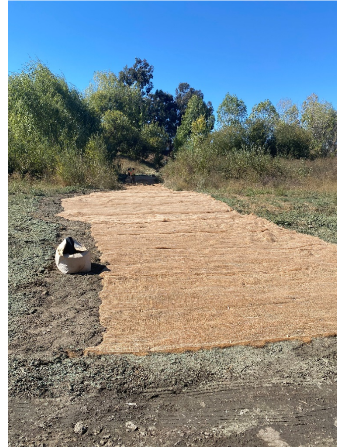
Access Road at Site #1 before and after w/hydroseed and erosion control mat
