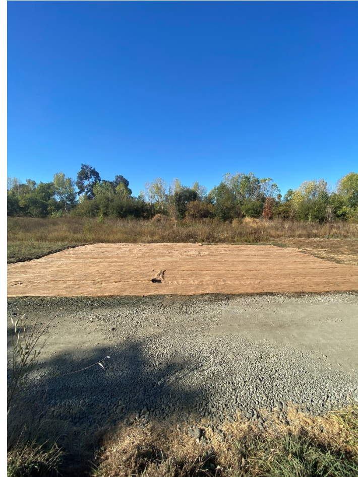
Staging Area – before and after w/hydroseed and erosion control mat
